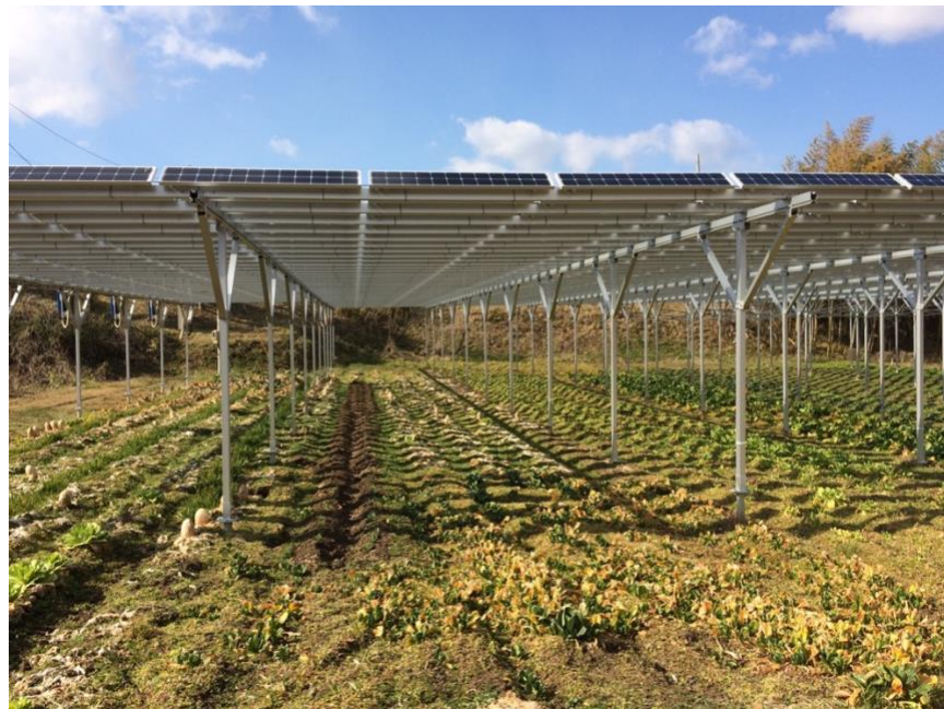
Figure 3.6: Solar sharing installation on cultivated farmland in Fukushima, Japan (photo by author).
