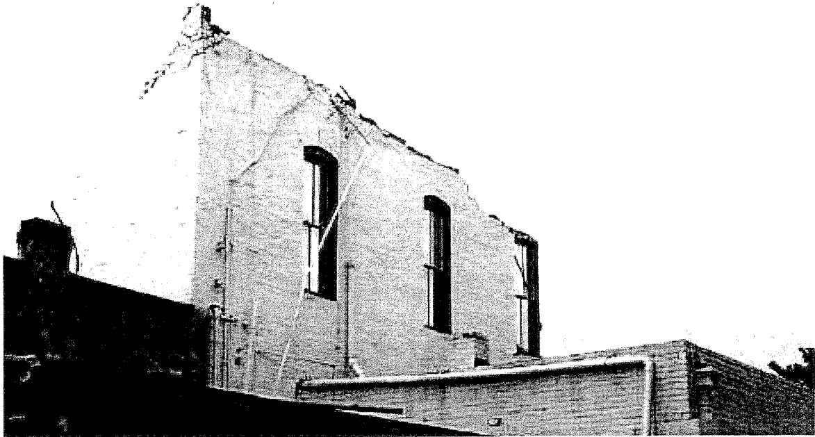
Figure 2: Part of a URM wall section that is still standing despite the collapse of the rest of the second story. December 22, 2003 San Simeon, California earthquake ( http://peer.berkeley.edu/san_simeonEQ/ ).
