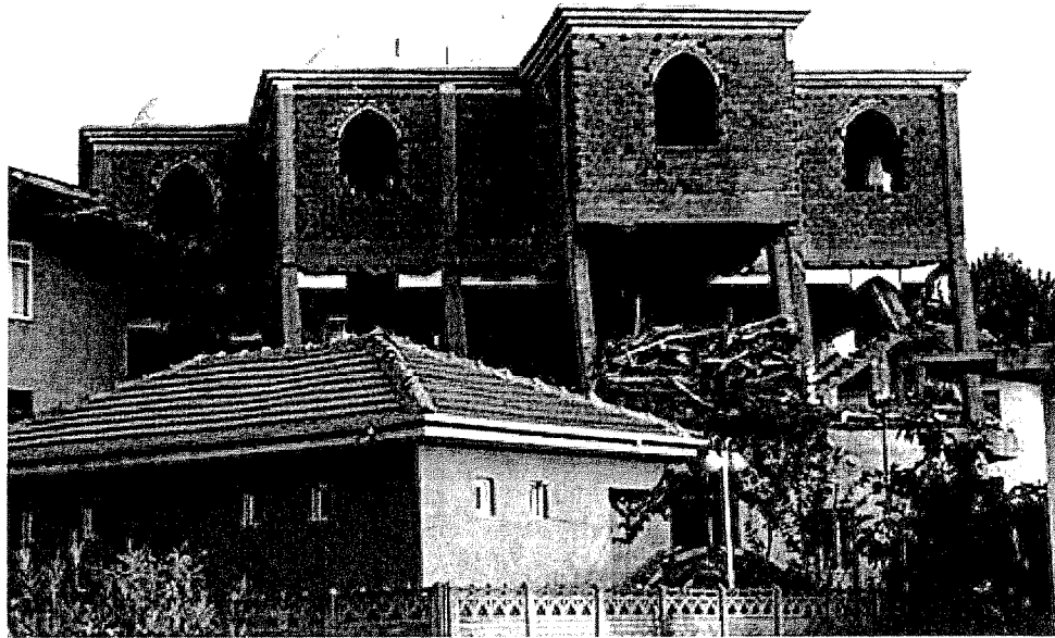
Figure 3: Reinforced concrete frame with collapse of brick infill and arched windows, August 17, 1999 Izmit (Kocaeli), Turkey earthquake ( http://nisee.berkeley.edu/images/servlet/EquisListQuake ).
