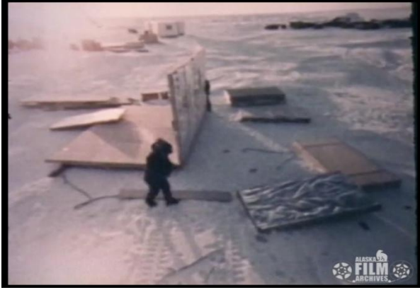
Fig. 11 | “Eskimo carpenters” constructing housing on an ice floe. From the NARL collection (AAF-233) at the Alaska Film Archives – University of Alaska Fairbanks.
