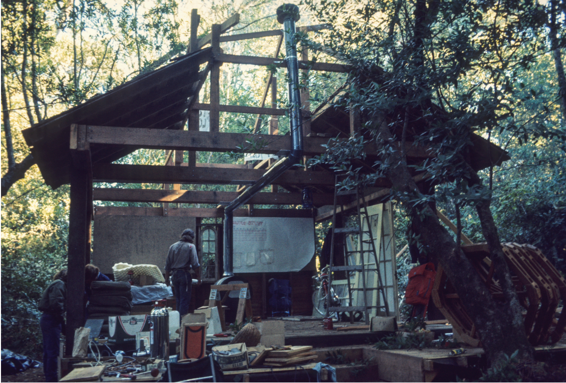
"The Arc" communal room and drafting studio under construction, UC Berkeley "Outlaw Builder Studio," Inverness, California, 1972. Photo courtesy of Jim Campe.
