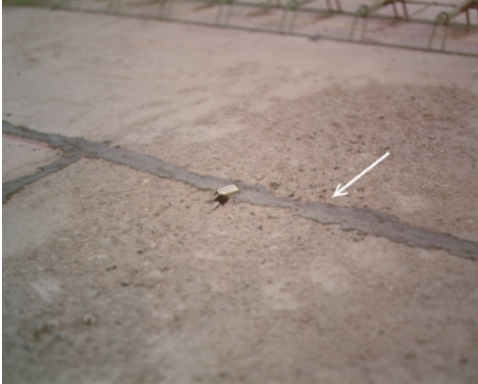
Figure 6.3. Backfilled Instrumentation Lead Channel on North Tangent CTB.
