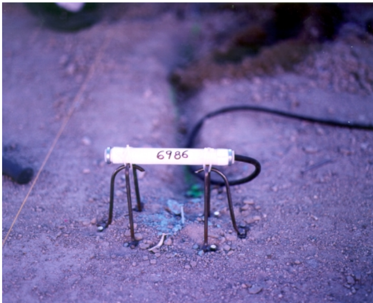
Figure 6.23. Carlson A-8 Strain Meter prior to Placement of Concrete, South Tangent.
