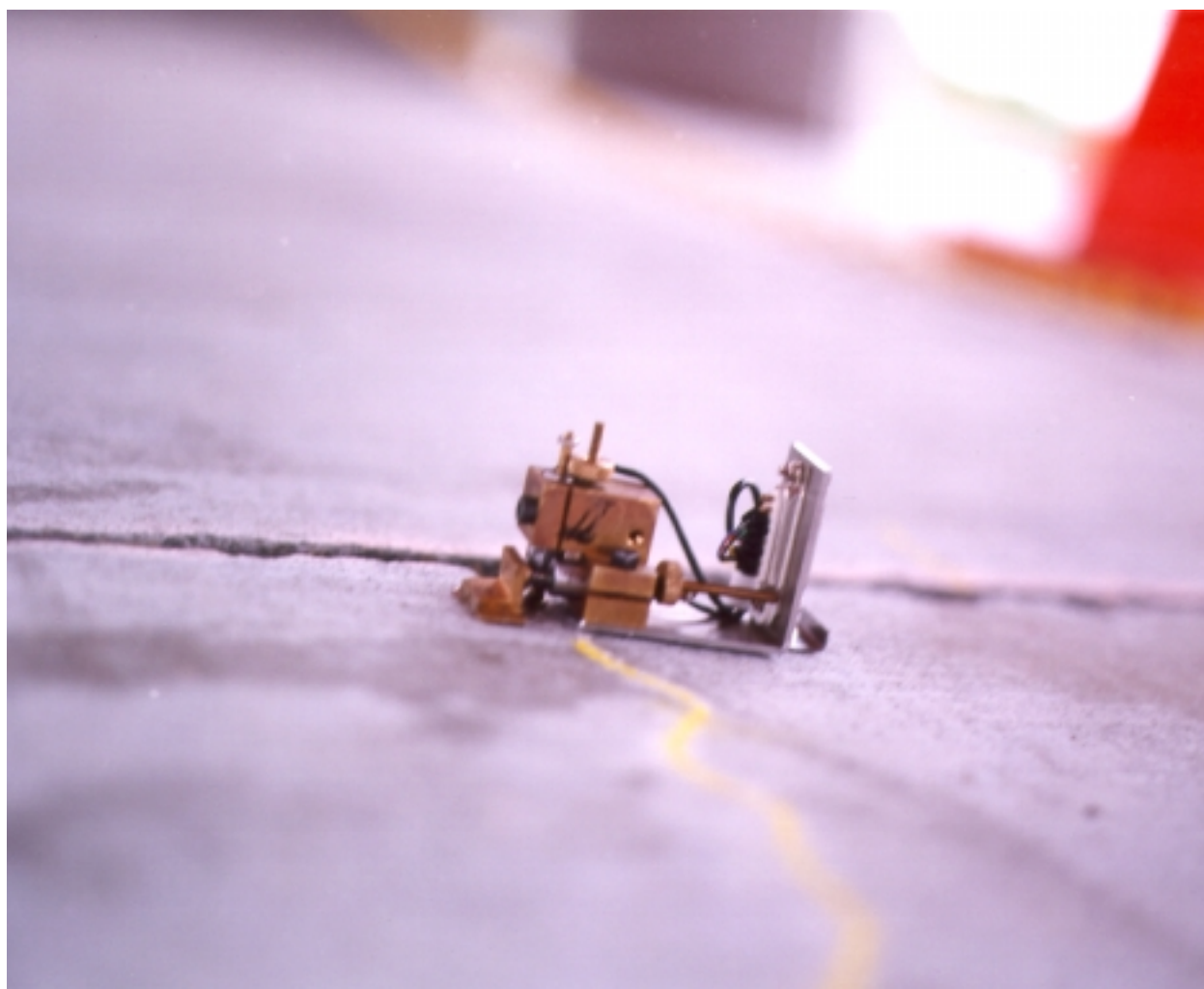
Figure 6.20. Crack Activity Meter (CAM) in Typical Position over a Crack.
