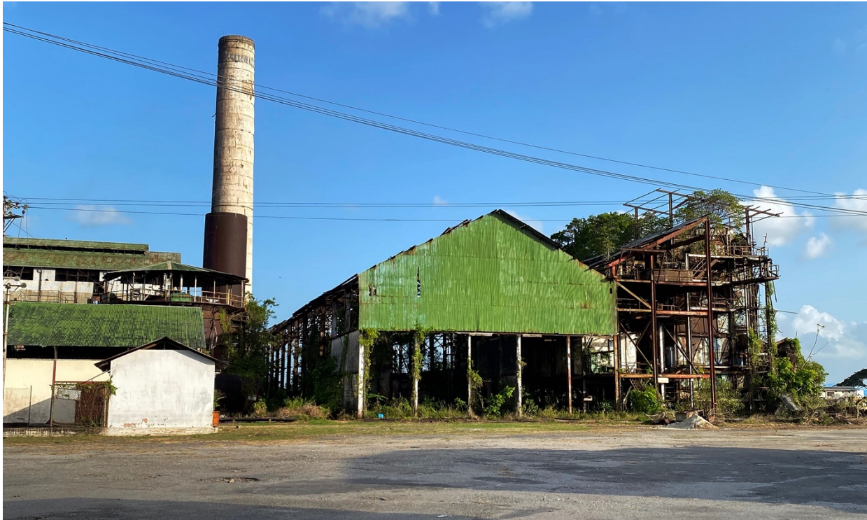
Figure 4. Abandoned sugar refinery in Couva, Trinidad, 2022. Photograph by Luis Vasquez La Roche.
