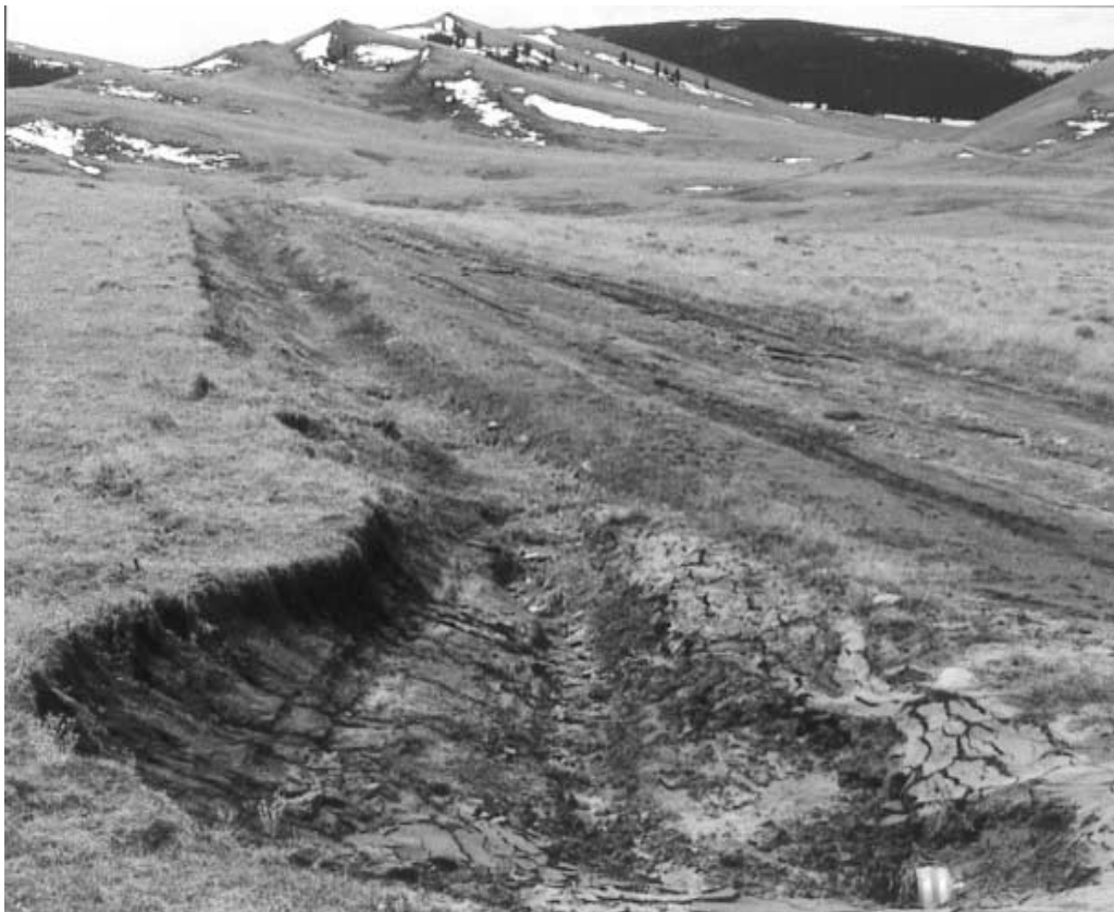
Fig. 2. Road damage resulting from lack of maintenance.
