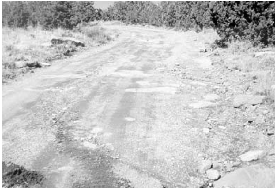
Fig. 6. A typical road section before in-place processing.
