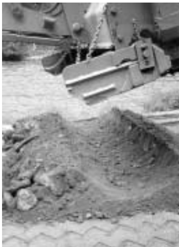
Fig. 4. Rotary drum processing a road surface.
