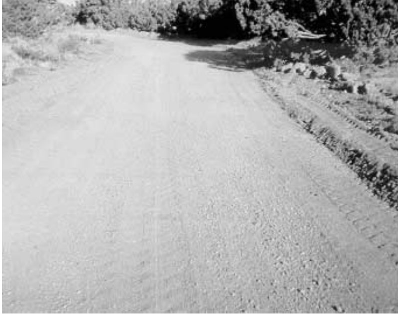
Fig. 7. A typical road section after in-place processing.
