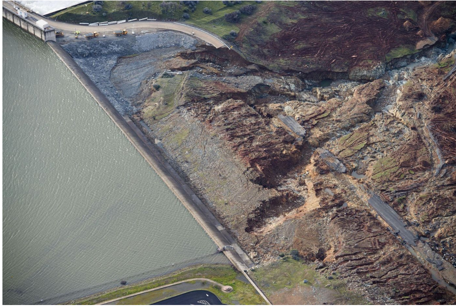
Figure 1.1: Erosion of the emergency spillway at Oroville Dam in Northern California, 13 February 2017 [82]
