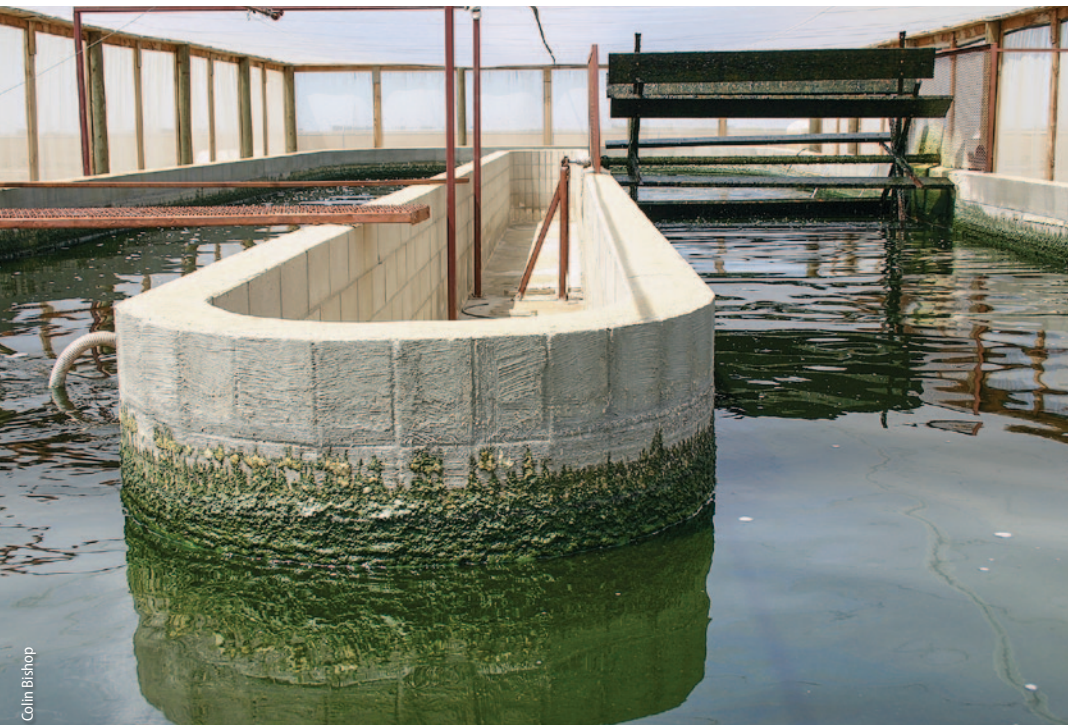
Water treatment facilities at San Joaquin Valley farms. Irrigation water high in nitrogen can contribute to growth of algal blooms, especially blue-green algae.
