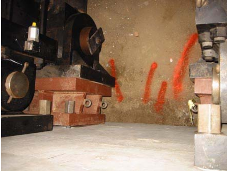
Figure 4.17. Soil cracking observed from above at 4 inches of head displacement.
