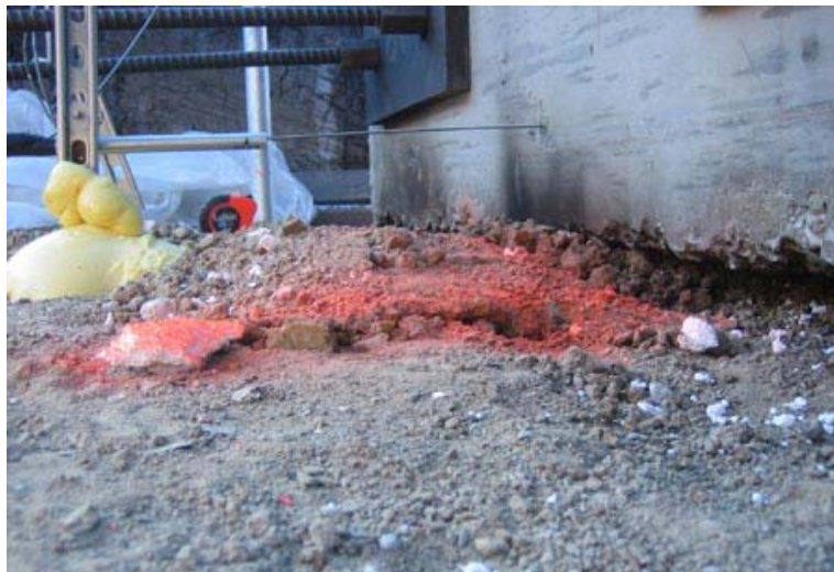
Figure 4.16. Heave and ground deformations observed at 4 inches of head displacement.
