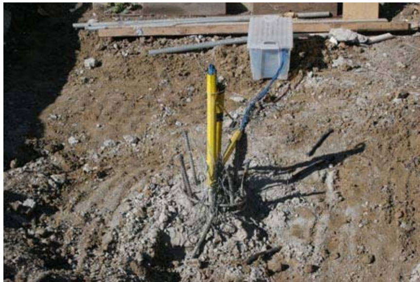
Figure 4.18. Investigation of longitudinal bars at the cap-shaft interface.
