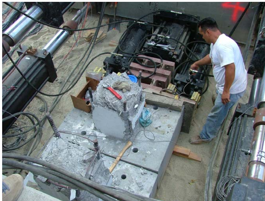
Figure 4.35. Installation of 3 supplemental actuators
