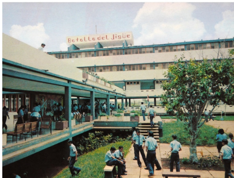
Figure 4.3. Above: Site plan of the typical rural boarding school indicating 1) access; 2) classrooms block; 3) open gallery corridor; 4) plaza; 5) kitchen-dining room; 6) dormitories block. Source: Ministerio de la Construcción, Josefina Rebellón's personal archive. Below: Informal gathering in the main corridor and plaza of the Batalla del Jigüe rural boarding school, as shown in a postcard issued by the Cuban government in 1972. The dormitories block is visible in the back. Source: author's personal collection.
