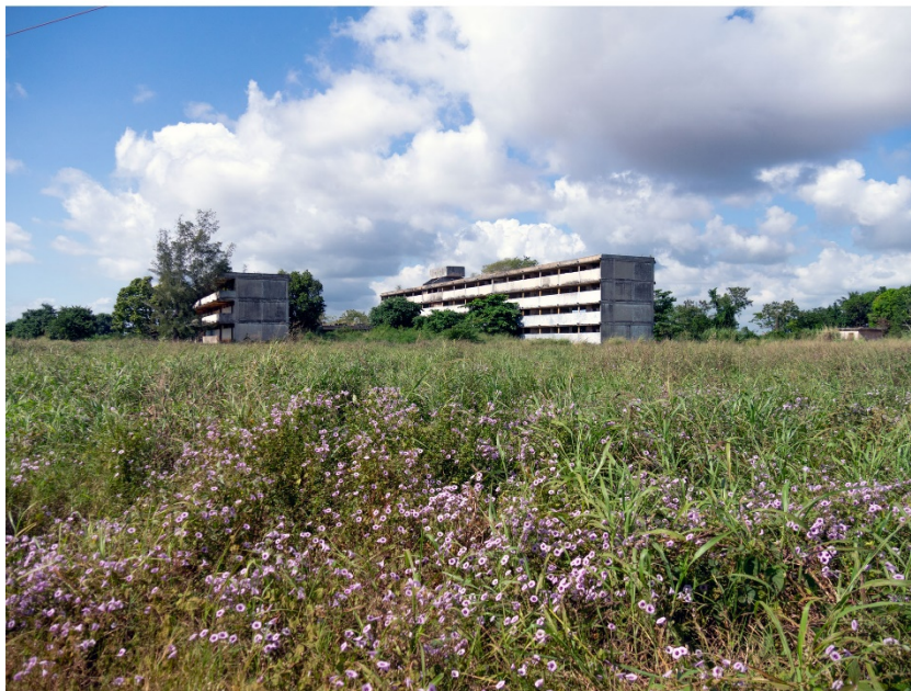
Figure 4.4. The two images illustrate the barrier-less connection between the typical rural boarding school building and its surrounding agricultural fields. Above: Taken from the second floor, this image shows the plaza's floor of a rural boarding school, now vacant, extending into the surrounding countryside. Below: This image of another rural boarding school, also vacant, shows how the agricultural fields become the plaza's fourth limit. The other three limits are the open gallery corridor (not visible in the photo), the classrooms block (left) and the dormitories block (right). Source: author, 2018.
