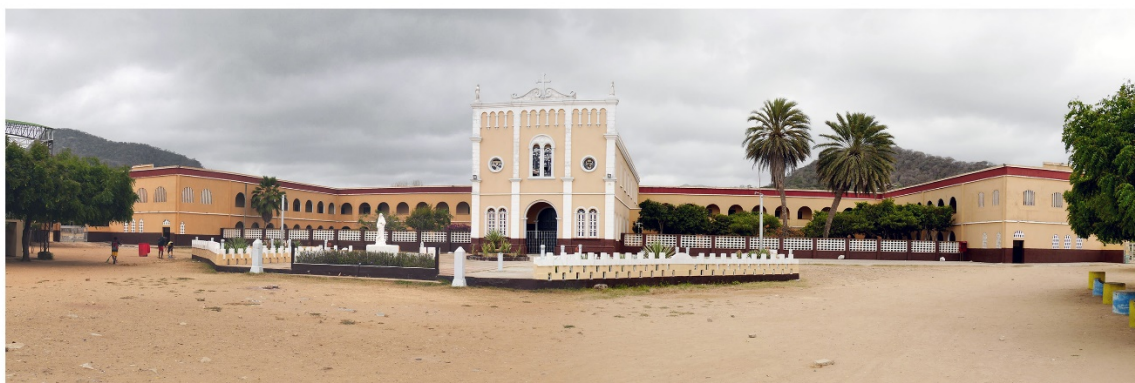
Figure 2.4. Above: Floorplan of Nazaret's boarding school in the early 1960s, based on the extant building and recollections from students. 1) chapel; 2) kitchen; 3) dining rooms; 4) monks' (left) and nuns' (right) rooms; 5) dormitories; 6) night guard's room; 7) classrooms. In red: connection between both sides not mediated by the chapel. Below: Nazaret's boarding school in 2018. Source: author.
