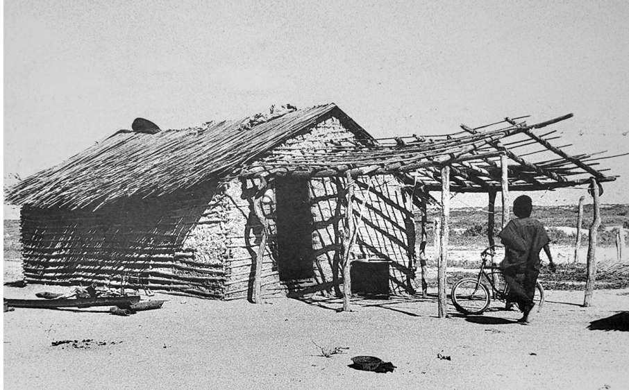
Figure 1.4. Typical Wayúu dwelling (still used today) with the luma (arbor) preceding the entrance (c.1990). Source: Lorenzo Fonseca and Alberto Saldarriaga, eds., Vivienda Guajira (Bogotá: Caribol, 1992).
