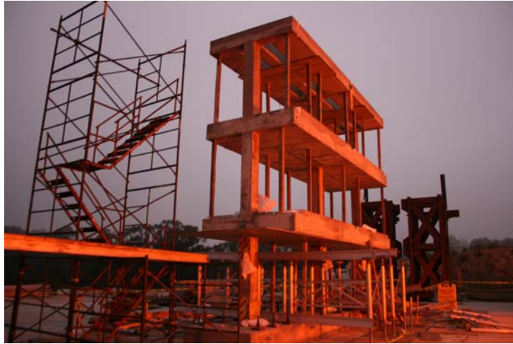
Figure C.22: Completed RC frame.
