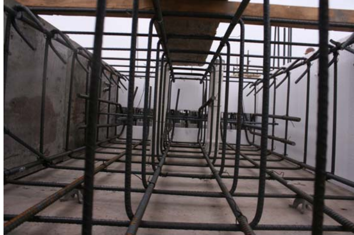
Figure C.16: Slab reinforcement and foam used to form concrete hinge.
