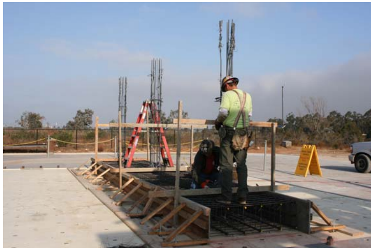
Figure C.8: Reinforcement and formwork for the foundation.
