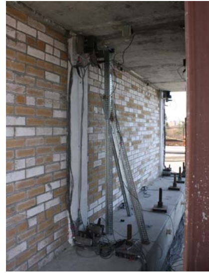
(b) pole installed at the first story
