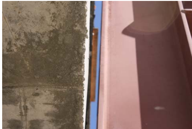
(b) gap between the specimen and the steel tower
