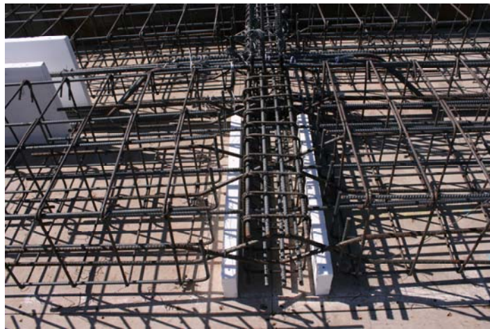
Figure C.11: Detail of first story beam-slab connection reinforcement.
