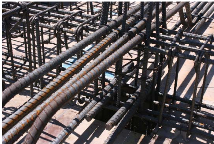
Figure C.15: Detail of middle column-beam reinforcement..
