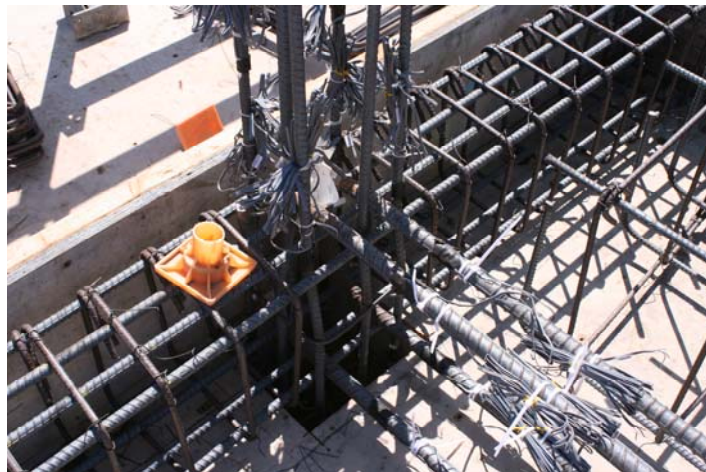
Figure C.12: Detail of joint reinforcement.
