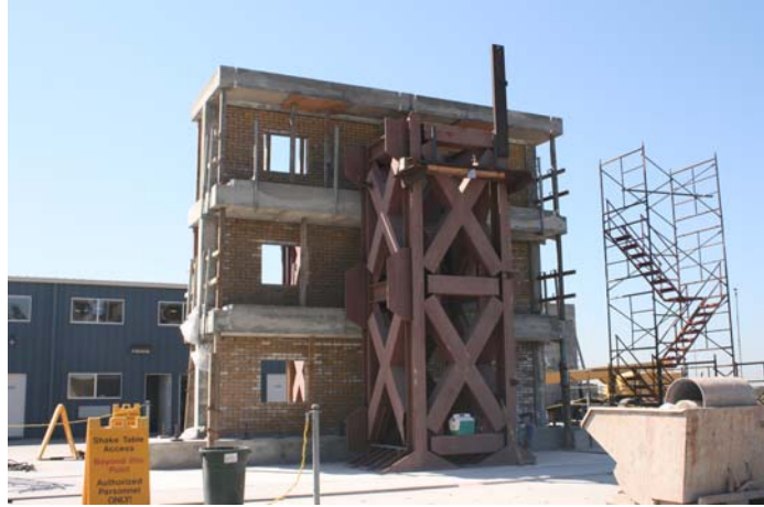
Figure C.28: Completed infilled frame.
