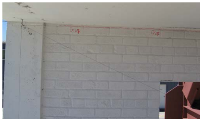
Figure D.14: Attachment of strings measuring the frame deformations (top of East column).
