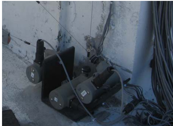
Figure D.13: String pots measuring the frame deformations (bottom of middle column).
