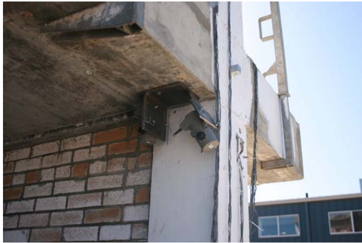
Figure D.12: String pots measuring the frame deformations (top of West column).
