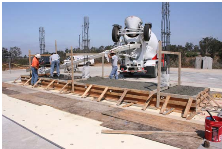
Figure C.9: Concrete pour for the foundation..
