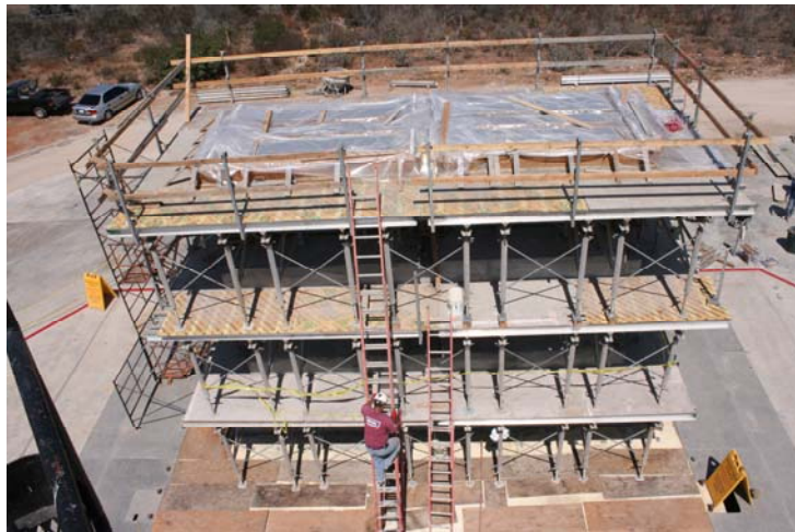
Figure C.21: Completed RC frame with form work.
