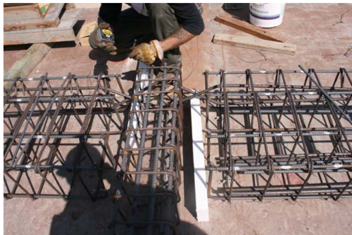
Figure C.18: Transverse beam and slab reinforcement.
