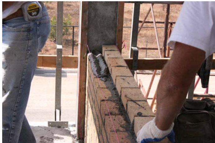
Figure C.29: Laying bricks with running bond.
