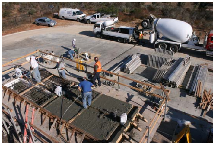
Figure C.14: Concrete pour for the first story columns, beams, and slabs.
