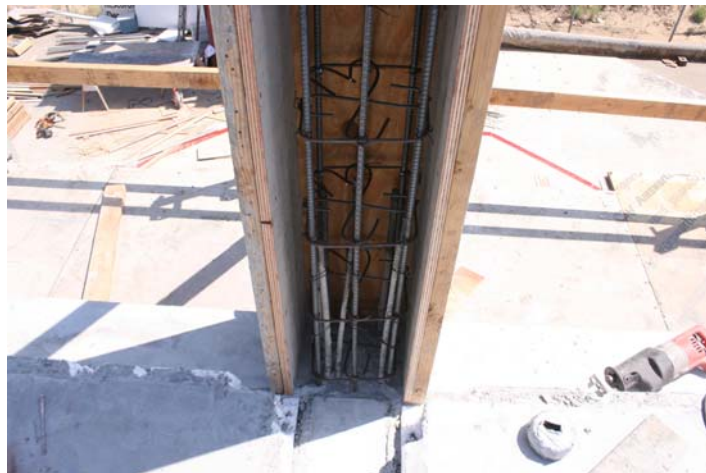
Figure C.17: Detail of column lap-splice.
