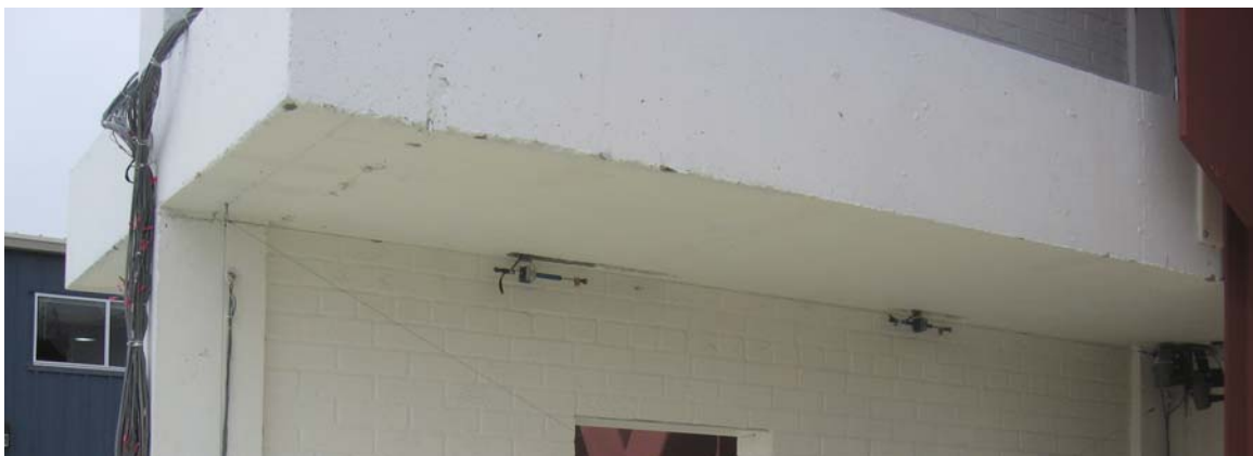
Figure D.6: LVDTs measuring the sliding of the infill wall with respect to the beam.
