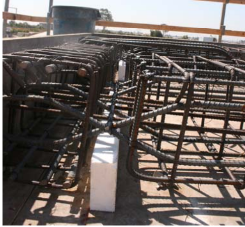
Figure C.19: Steel reinforcement and foam used for slab-to-beam connection.
