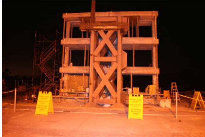
Figure C.25: First bay almost infilled.
