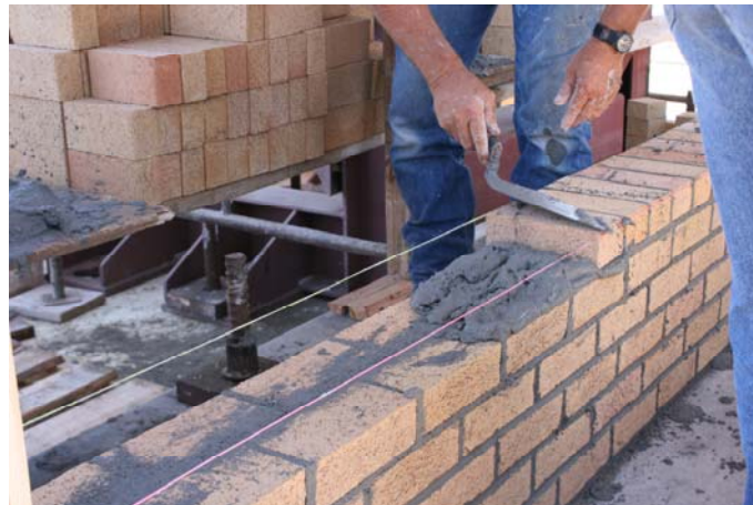
Figure C.24: Laying the head course.
