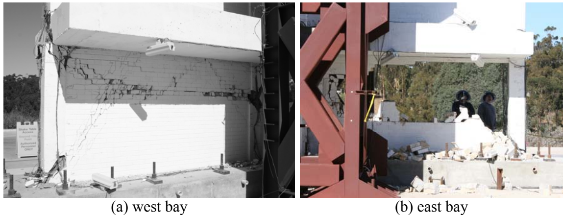
Figure 9.38: First story panels after ec250.
