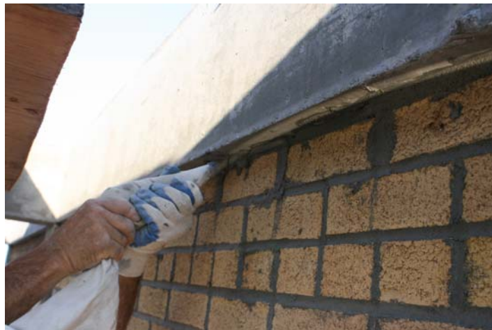
Figure C.26: Dry-packing of beam-to-infill wall.
