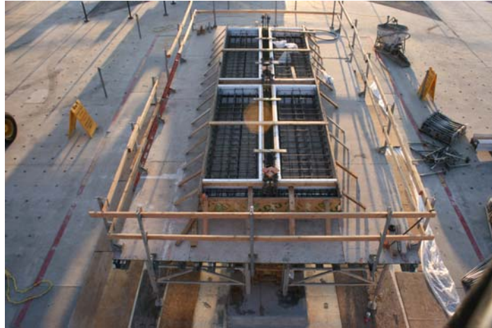
Figure C.13: First story beam and column reinforcement.
