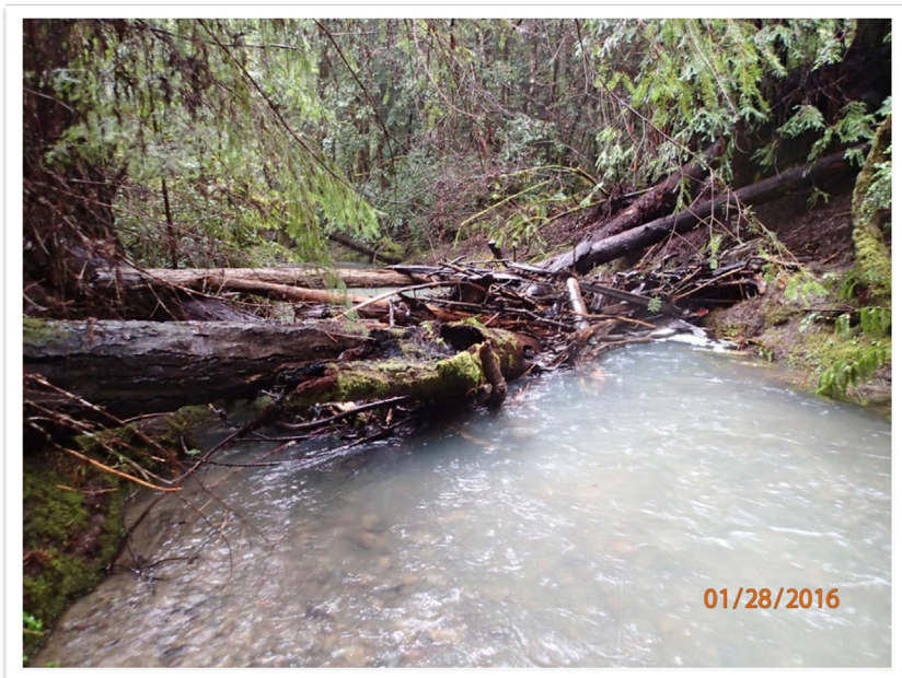
Figure 7. Additional woody debris collected by the structure shown in Figure 6 after the first winter in an active stream channel. Photo credit: Alan Ader, California Conservation Corps.
