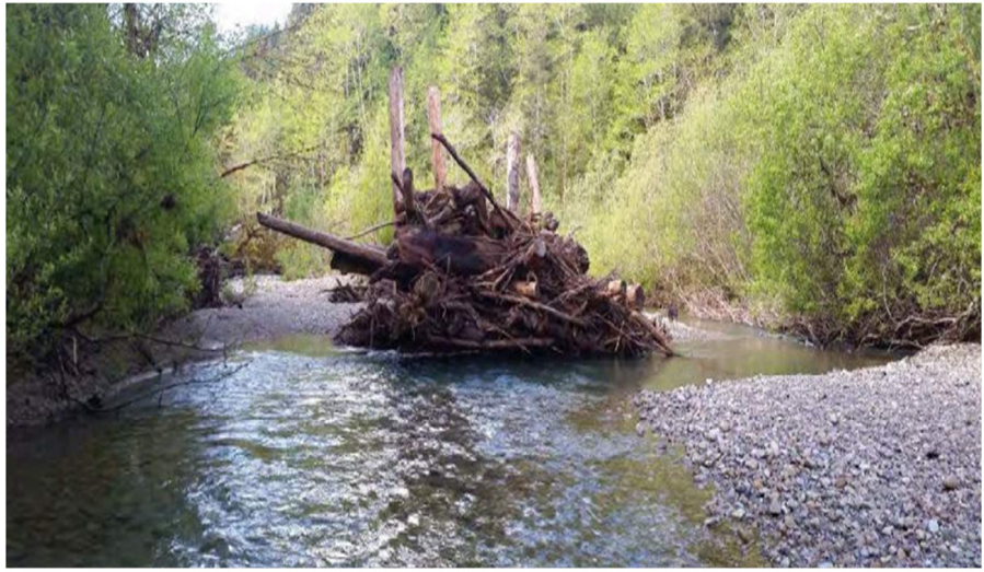
Figure 13. Apex bar jam. Photo credit: Rocco Fiori, Fiori GeoSciences.
