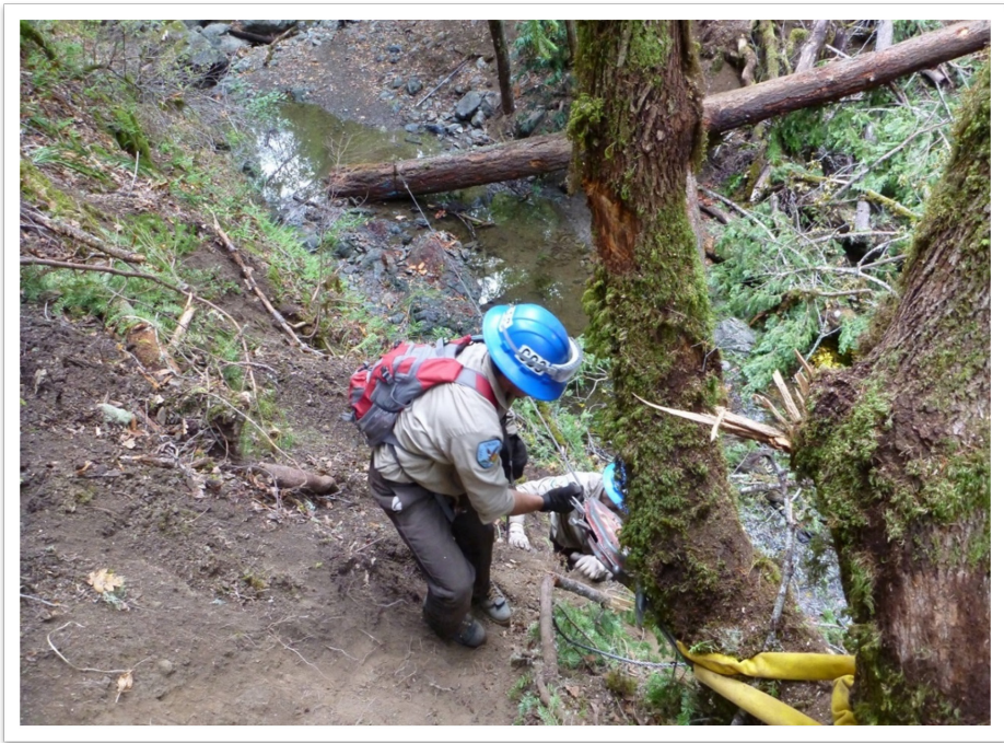
Figure 15. California Conservation Corps member moving a log with a portable lever operated hoist. Photo credit: Derek Acomb, CDFW.
