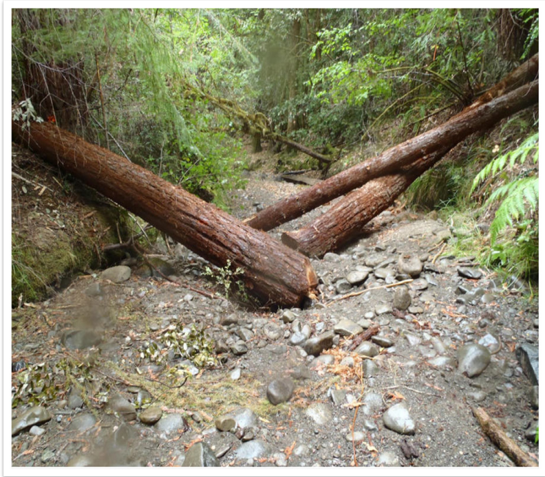
Figure 6. Logs placed at an upstream angle against the banks of a dry stream channel. Photo credit: Alan Ader, California Conservation Corps.
