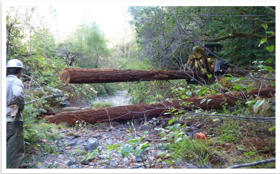
Figure 14. Placement of logs from the streambank using a rubber-tired grapple skidder. Photo credit: Derek Acomb, CDFW.
