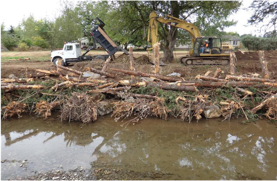
Figure 28. Vertical logs used for weaving angled logs rather than for structural stability. Photo credit: Clackamas Soil and Water Conservation District.
