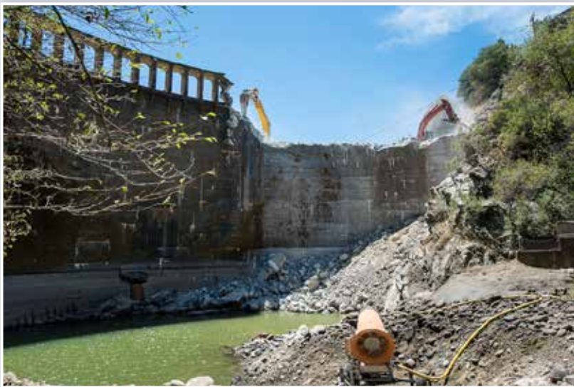
Demolition of the 106-foot-high San Clemente Dam on the Carmel River. Photo: California American Water
