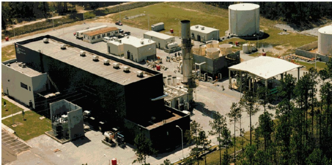
Figure 10: Aerial View of CAES Plant in McIntosh, Alabama
