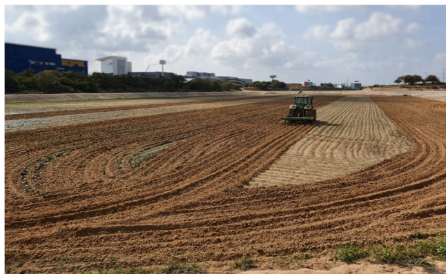
Fig. 4. Tillage in a soil aquifer treatment (SAT) infiltration basin in the Israeli Dan Regional Reclamation Project (Shafdan).
