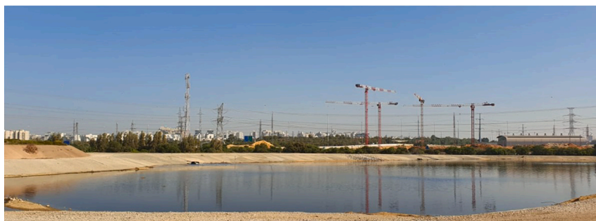
Fig. 3. Soil aquifer treatment (SAT) infiltration basin in the Israeli Dan Regional Reclamation Project (Shafdan) during the wet cycle. Note the nearby construction in the background, illustrating the need for alternative land areas.
