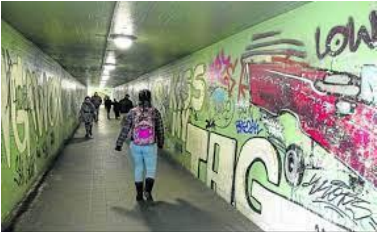
Figure 27. Pedestrian tunnel in Valladolid.
