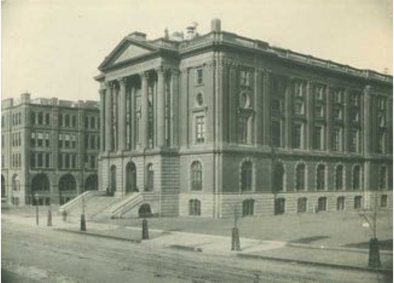
Figure 7. Rogers Building (1866), Massachusetts Institute of Technology. Courtesy of MIT Institute Archives and Special Collections.
