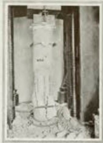
REINFORCED CONCRETE COLUMN View showing a concrete column with vertical steel rods after failure. The top of the column is covered with an iron plate imbedded in plaster of Paris to insure an even bearing. A load of 400,000 pounds produced failure.
