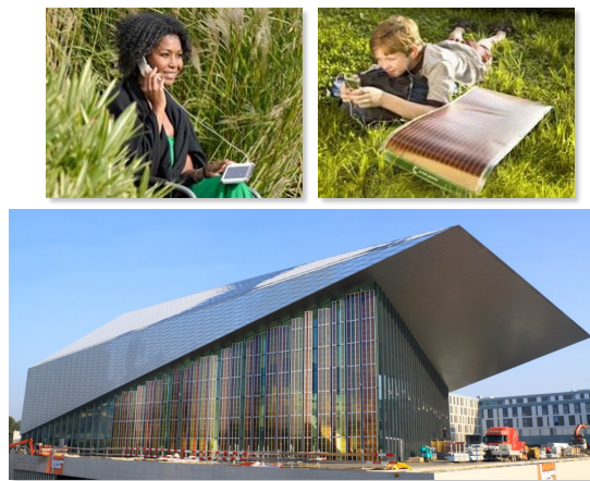
Figure 1.2: DSSC uses in real life (Top) G24:solar charging for mobile devices (from [1]) (Bottom) Solaronix' multicolored transparent photovoltaic facade at the SwissTech Convention Center, EPFL, Switzerland (from [19]).
