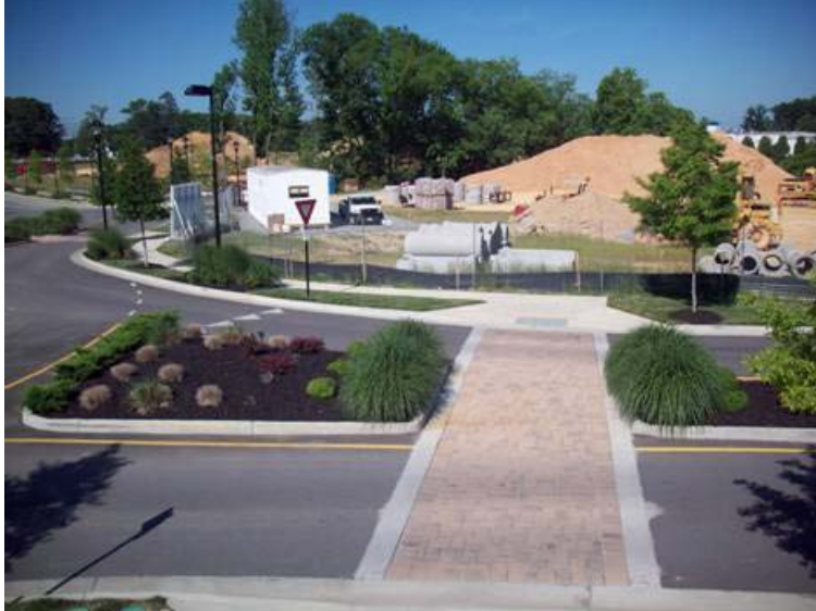
Figure 8: Landscaped Splitter Island on Roundabout Approach Henrico County, VA
