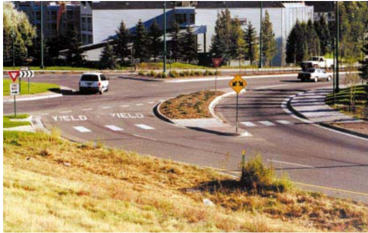
Figure 21: Example of a Right-Turn Bypass Lane with a Yield at Exit Leg (FHWA Guide)
