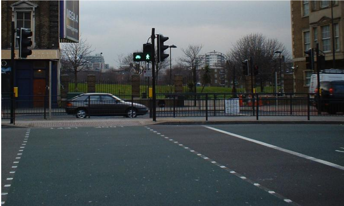
Figure 28: Toucan Crossing at Roundabout in England
