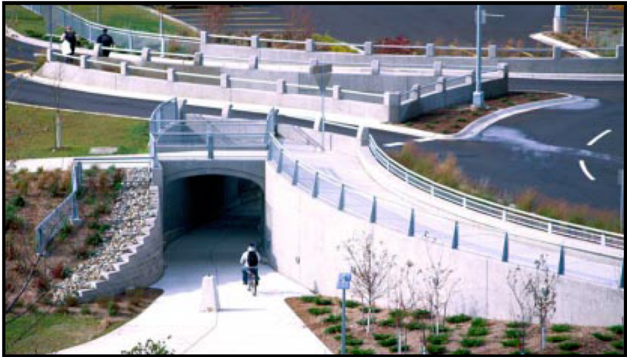
Figure 22: Bicycle and Pedestrian Roundabout Undercrossing at Western Michigan University
