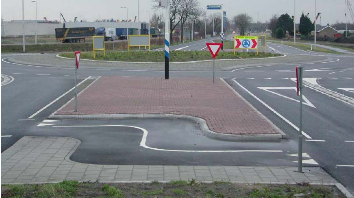
Figure 27: Jog in bicycle path on splitter island
