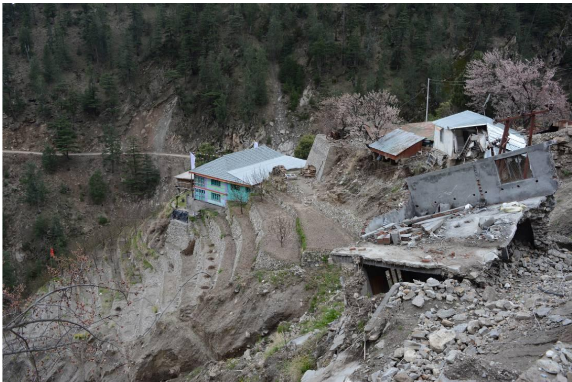
Figure 7: Destroyed buildings and apple orchards from landslides during the 2013 monsoon season, Middle Kinnaur
