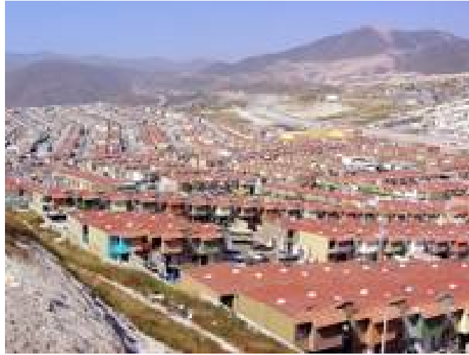
Figure 5. New Housing Developments in Tijuana
