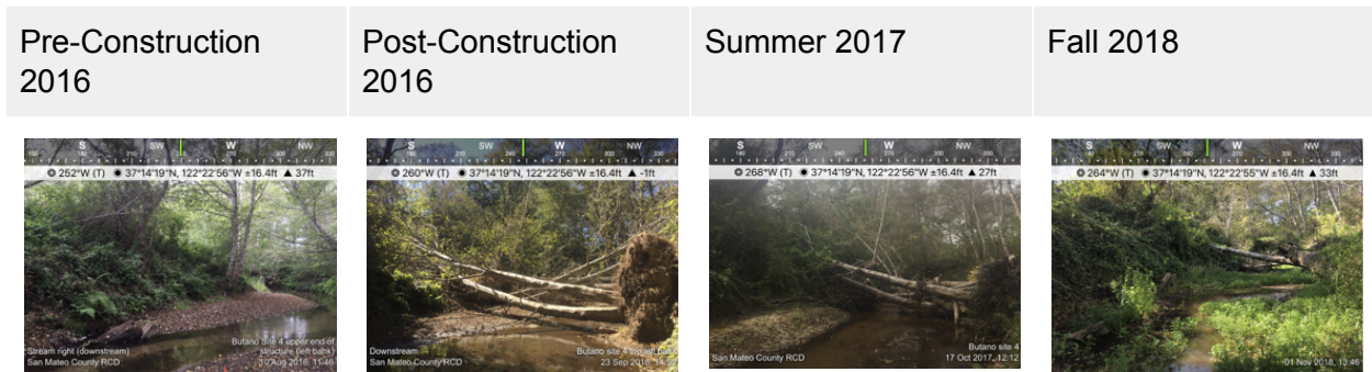
Figure 14: Butano Creek Site 4
