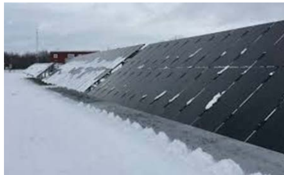
Figure 71. Frameless modules in the foreground and framed modules in the background: Both at a high tilt angle to allow snow to slide off. Source: DOE 2017.
