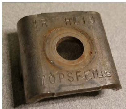
Figure 14. Clamping bracket: evidence of flange nut scrapes from loosening. Source: G. Robinson, LBNL.
