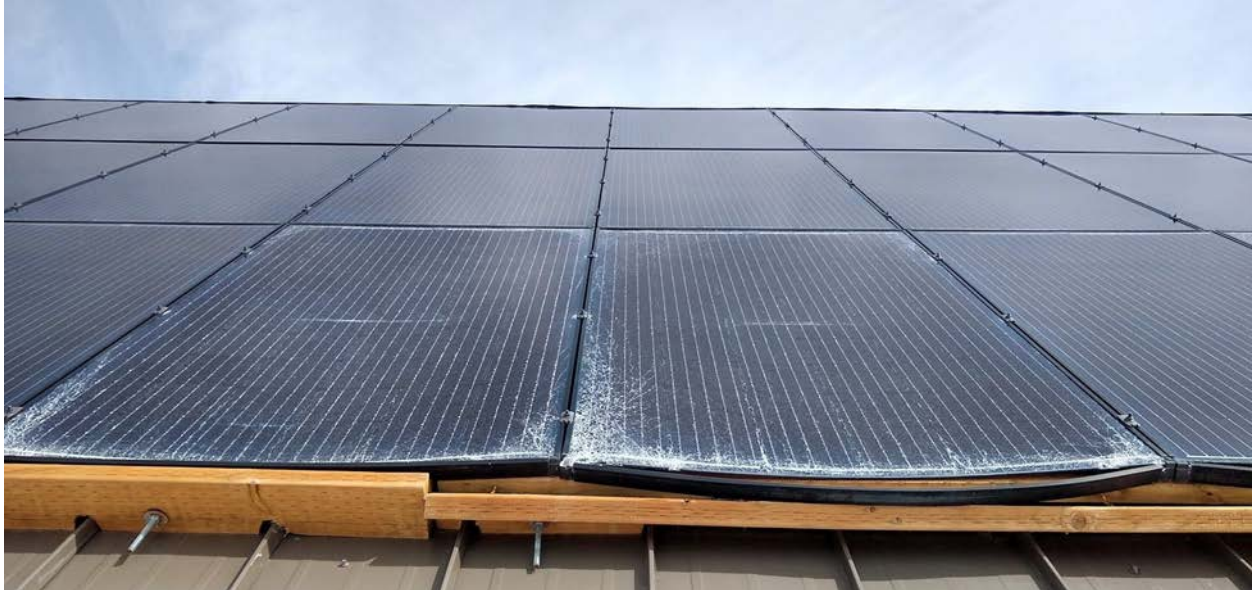
Figure 74. Modules damaged by snow at Sunrise at Mount Rainier National Park. Photo: Aaron Bougie, NPS.
