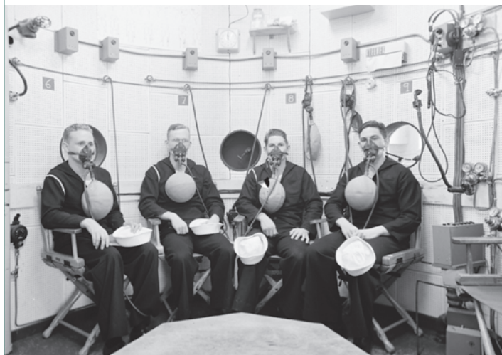
In this 1943 photo in the Donner Lab altitude chamber, four sailors breathe a mixture of radiolabeled gases to help determine how to protect pilots flying at high altitudes.
