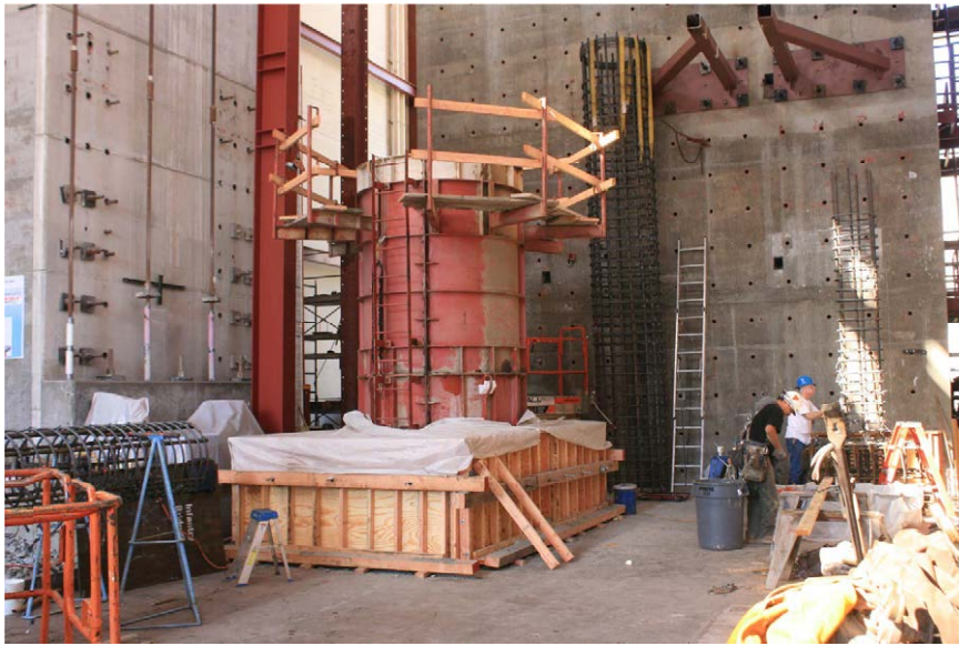
Figure B.7: Steel form for the shaft
