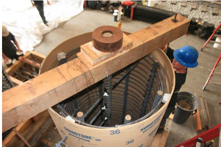
Figure A.4: Installation of the central bar
