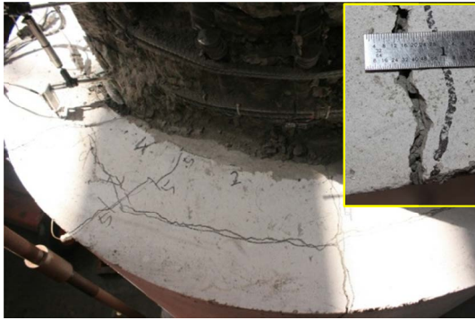
(c) Top of the shaft (north side)
