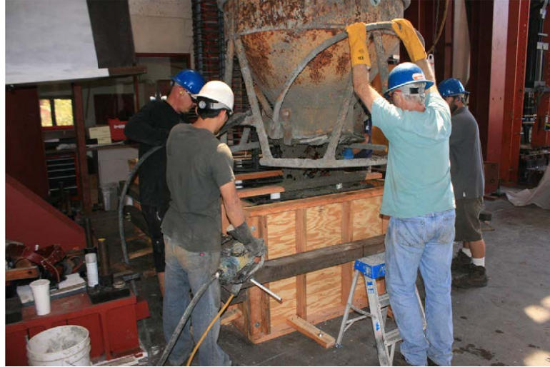
Figure A.2: Concrete pour of the footing
