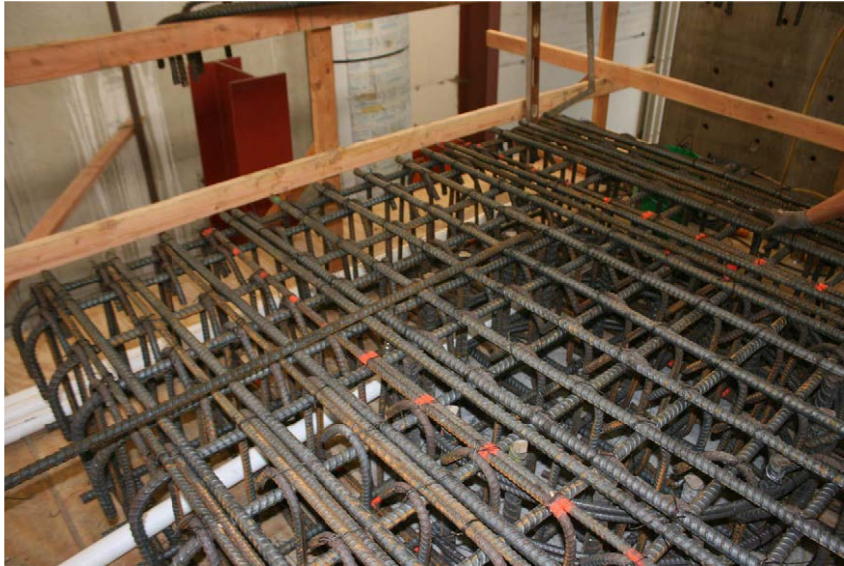
Figure B.17: Load stub reinforcing cage
