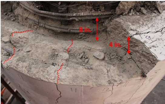
(c) Post-test inspection (Top of north face)
