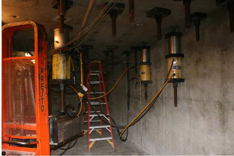
Figure B.25: Setup of hydraulic jacks under the strong floor to control the load of the vertical rods
