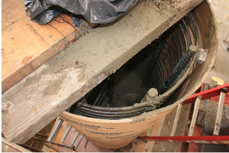
Figure A.6: Concrete pour of the cylinder
