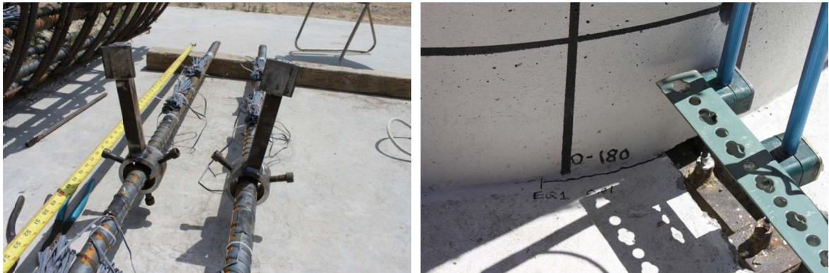
(a) steel pieces attached to column bars
