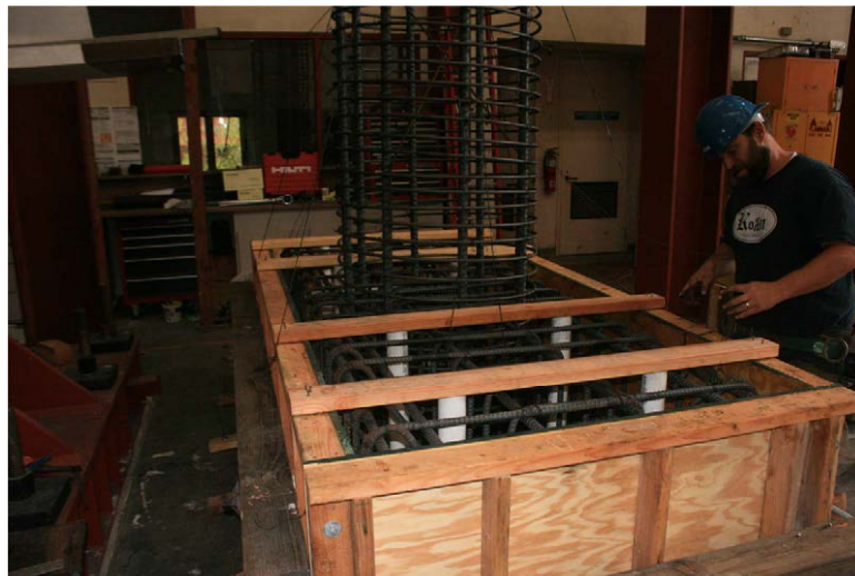
Figure A.1: Footing and cylinder cages and footing form
