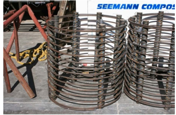
(b) Assembling steel cages and placing strain gages on spiral
