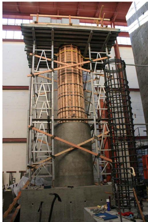
Figure B.14: Column form and falsework for load stub
