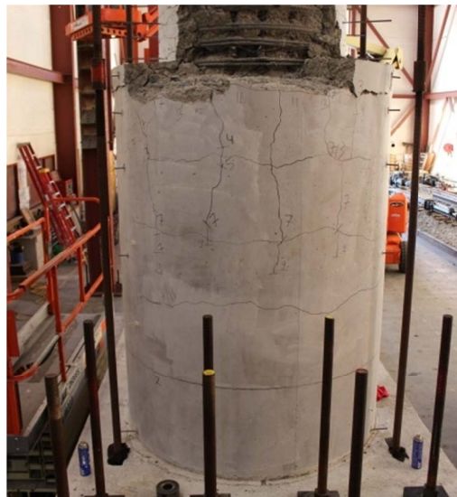
(e) Post-test inspection (north face)
