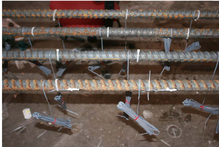
Figure B.1: Strain gages on longitudinal reinforcing bars
