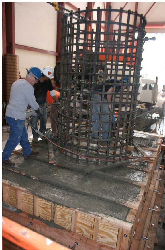
Figure B.6: Concrete pour of the footing (Pour 1)
