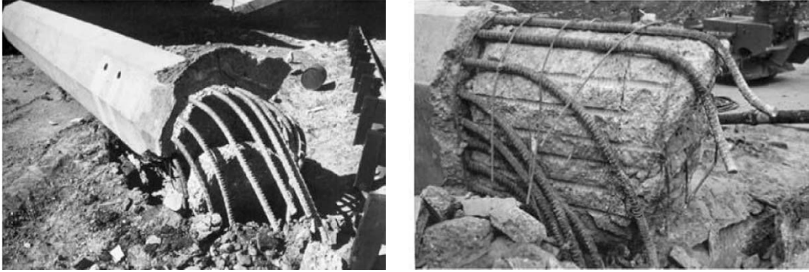
Figure 1.1: Pull-out of longitudinal reinforcement in bridge columns from foundations during the 1971 San Fernando earthquake (Yashinsky 2001)
