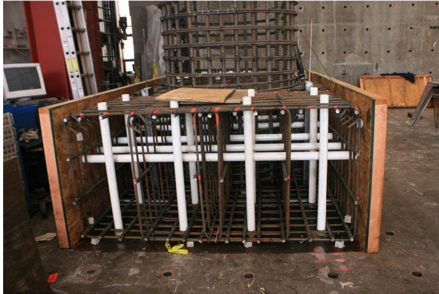
Figure B.5: Footing and shaft cages
