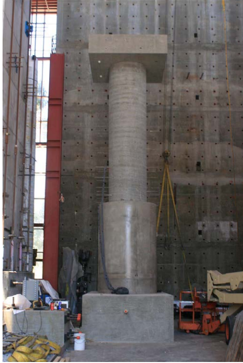
Figure B.19: Column-shaft after removal of the form and falsework
