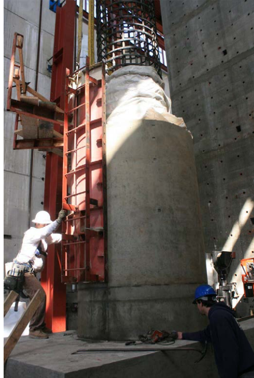
Figure B.13: Removal of the shaft form
