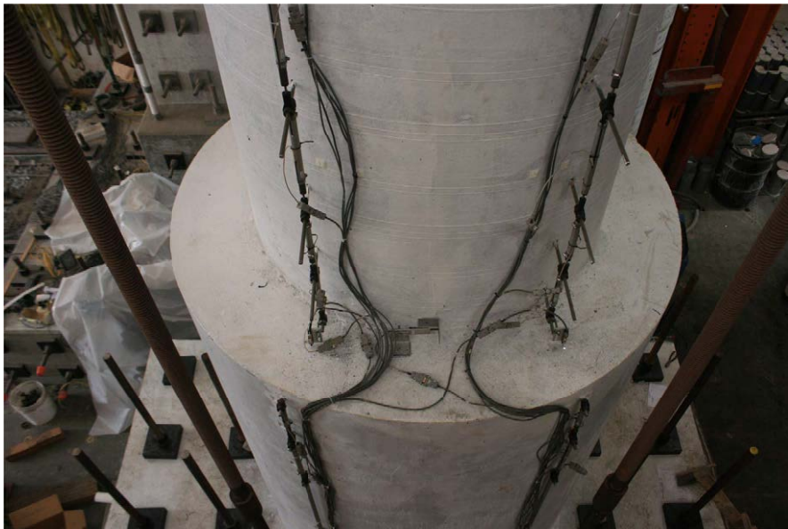
Figure B.22: Displacement transducers at the base of the column (east side)
