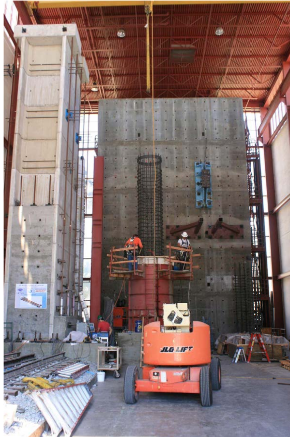
Figure B.11: Installation of the column cage
