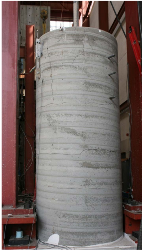
(a) splitting and circular cracks in the concrete cylinder
