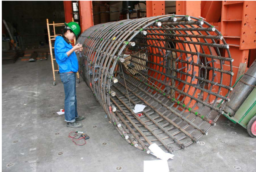
Figure B.3: Shaft cage instrumented with strain gages
