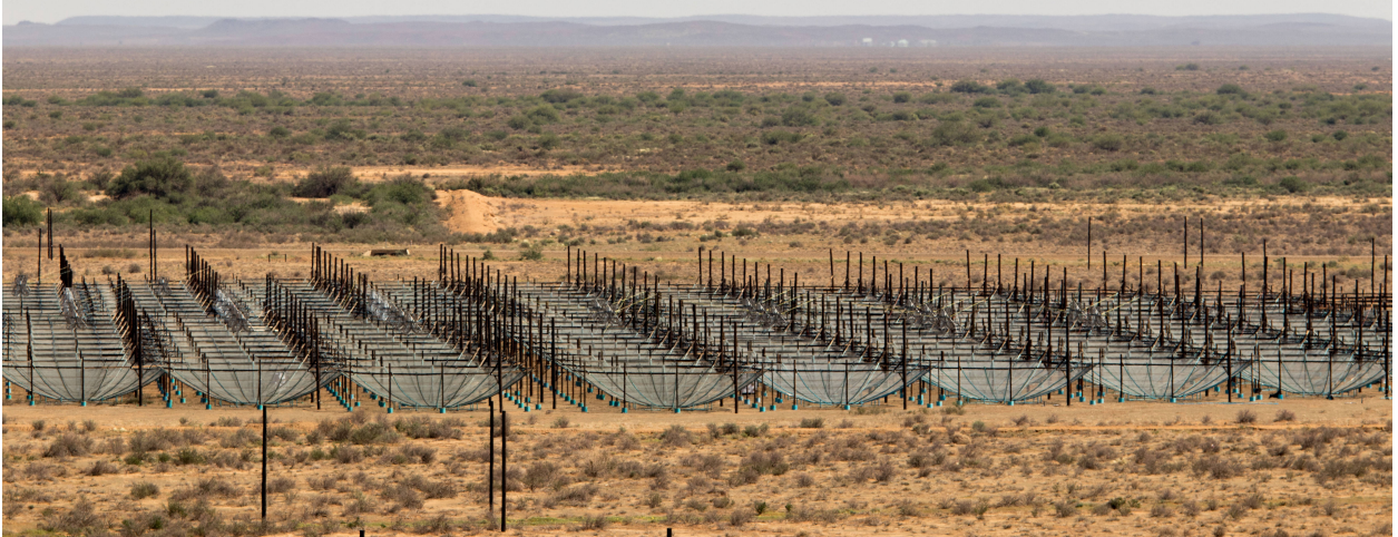
Figure 1.18: The Hydrogen Epoch of Reionization Array under construction in the South African Karoo Radio Astronomy Reserve. The antennas are 14.6 m diameter non-tracking parabolic dishes supported by wooden poles and built out of PVC pipes. Each antenna has a Vivaldi feed that can observe in the frequency range 50–250 MHz. The image shows 200 of the planned 350 antennas that are currently being commissioned for early science.
