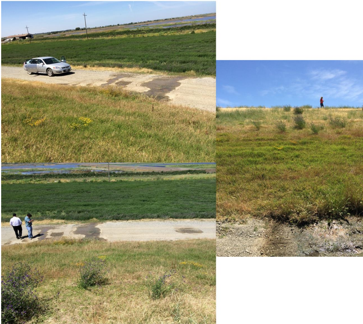
Figure 62: Field photos (by Cathleen Jones, JPL) of an active Seep #5 on Twitchell Island in June 2014.
