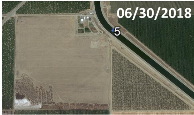
Figure 26C: Seep 5– Google Earth Imagery
