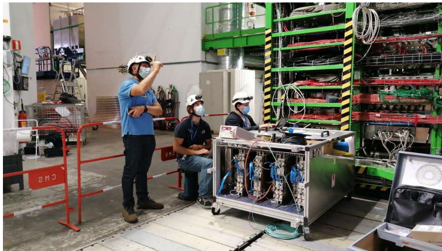
Figure 6.21: The setup of the “Trolley” Test inside the CMS cavern. The trolley contains the GE1/1 chambers; on top of the trolley is a bench top power supply to provide LV for the test. In the photo, Michele Bianco (left) is pointing out the GEM installation to the author (center) and Johny Jaramillo (right) while the trolley test is being performed.
