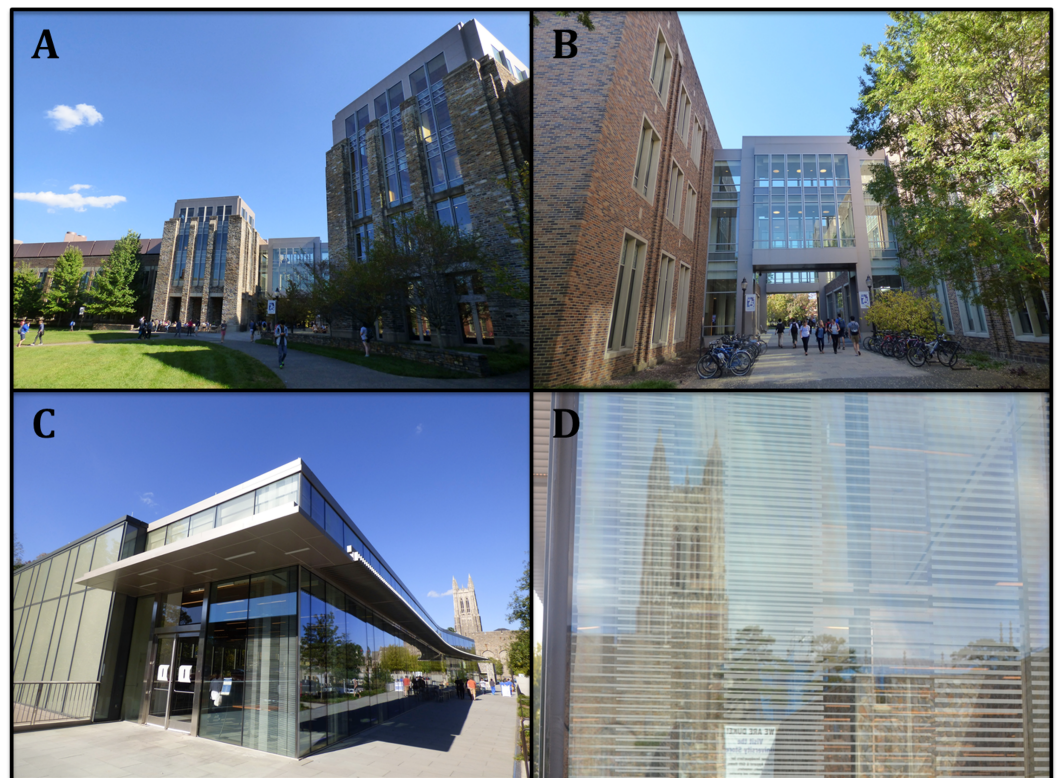
Figure 3 (A–B), Fitzpatrick, the buildings with the highest bird-window collision frequency at Duke University. (C–D) Penn, the only building with bird deterrence patterns at Duke University.
