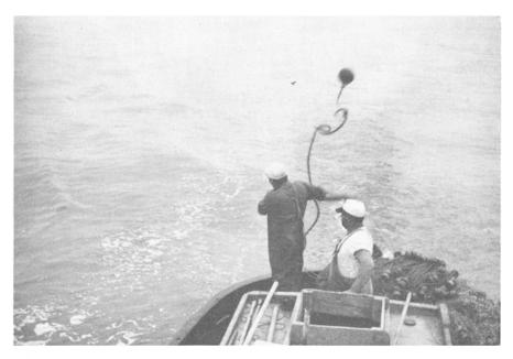
Figure 92. Fishing for bait with a lampara net. A weighted float attached to one end of the net is thrown from the boat, the boat moves continually in a circle as the net is payed out and the ends of the net are brought together at the float encircling the fish. Photograph by R. D. Collyer, August, 1948
