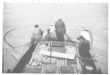
FIGURE 93. Pulling in the net. The bait is trapped between the walls of the net, and will be brailed into the opening of the bait tank (center of photograph) and held there until sold. Photograph by R. D. Collyer, August, 1948
