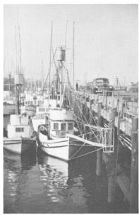
FIGURE 41. Typical swordfish boat showing plank, crows nest and trolling poles. Complete engine controls are extended to the crows nest. The trolling poles are vertical on either side of the crows nest and in trolling they are lowered to about a 30° angle above the horizontal. Photograph by Edward C. Greenhood, 1948
