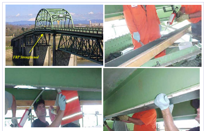
Figure 22: Field application of the h-lam system for the sauvie island bridge, Portland, Oregon, USA.
