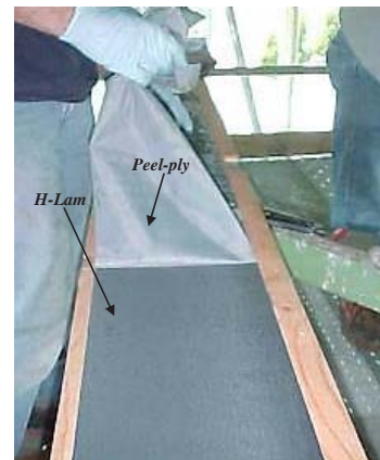
Figure 19: The H-Lam peel-ply.
