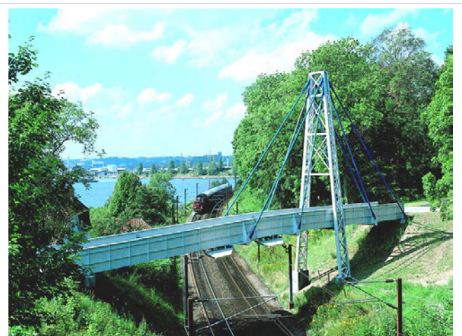
Figure 41: The fiberline all-composite cable-stayed in Denmark.
