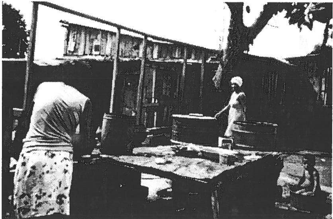
Illegally subdivided property in Gama, 1988
