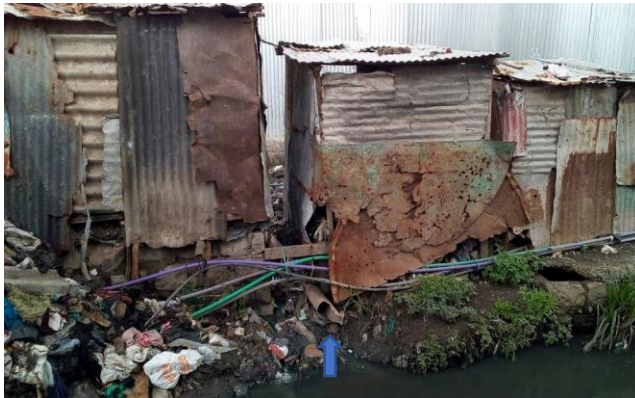
3) Drain directly to river (see pipe)
