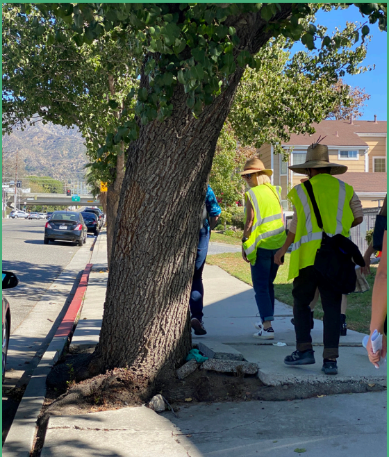
Figure 5. Insufficient tree well size
