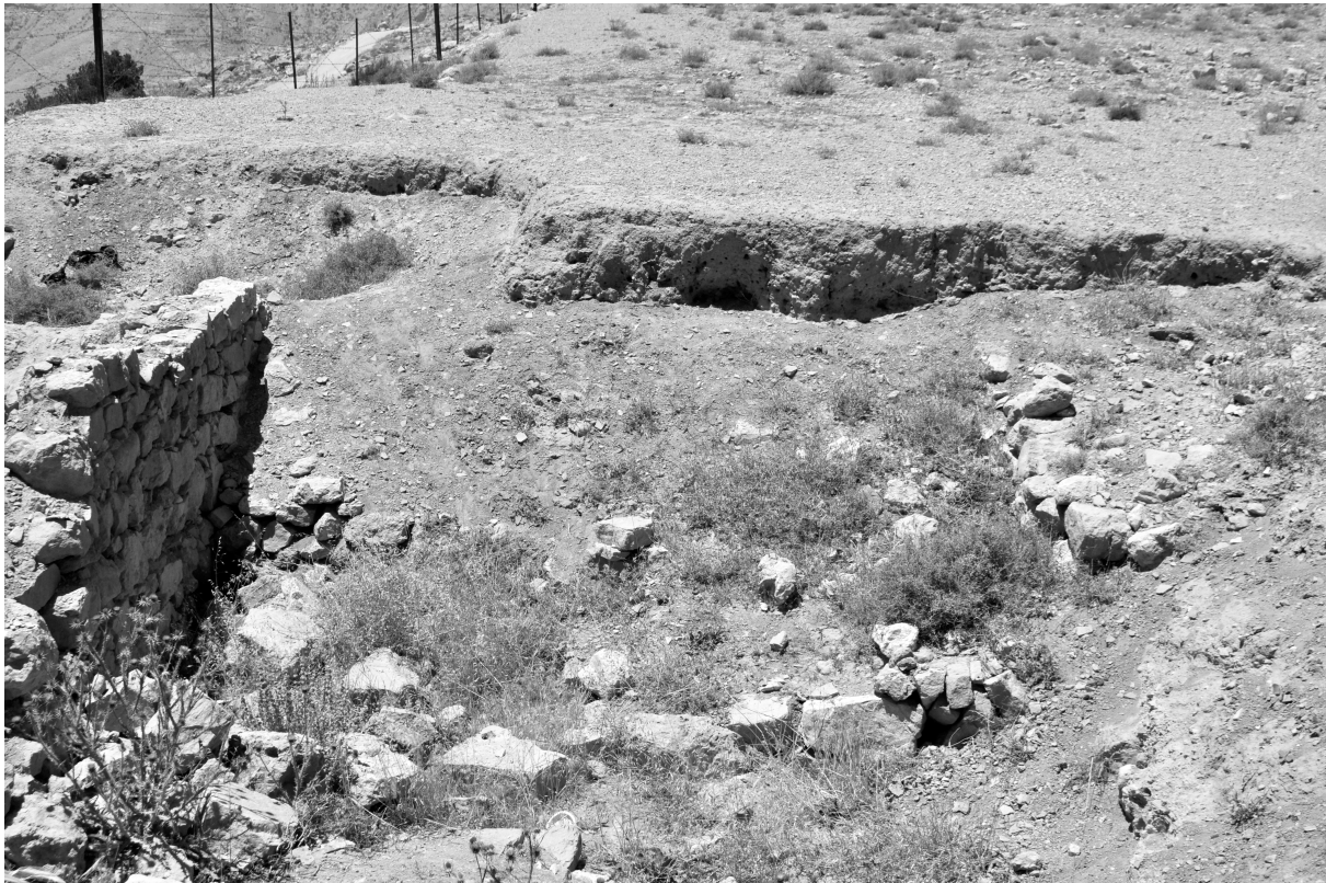
Figure 3. Collapse and erosion of west section in Area B near the postern gate (Image: B.W. Porter).
