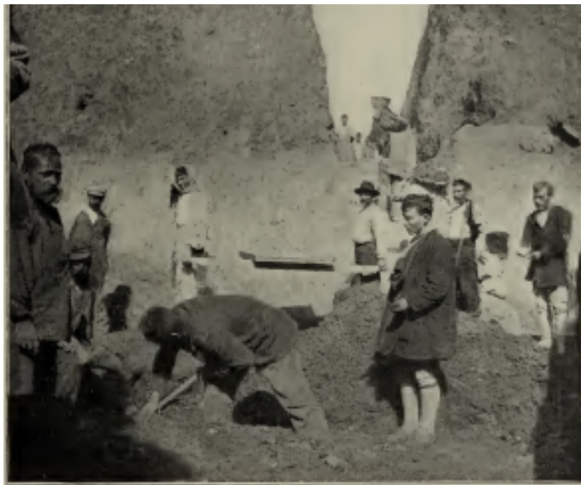
Figure 4.2: Excavation of Chaironeia Tumulus. Cooley 1904, 141.
