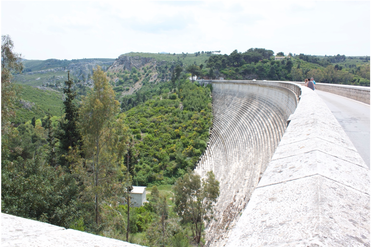
Figure 2.27: View from top of Marathon Dam. Notice stairs and path down from dam, inaccessible in 2019. Photo: Author.
