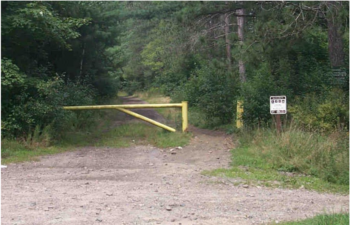
Figure 13. Gates used by the National Park Service often allow foot traffic while denying vehicle traffic.
