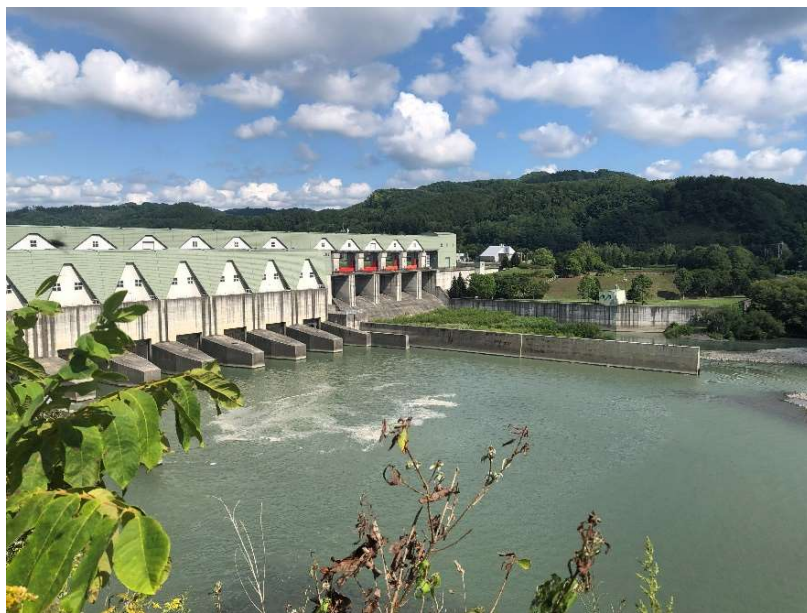
Image: A view of the Nibutani Dam from downstream.
