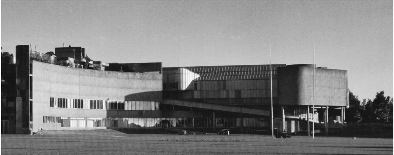
Figure 4.27 UCT Sport Centre, 1977. The design epitomizes the brand of modernism Uytendogaardt produced in Cape Town, that was humanistically responsive to the site and human body, while maintaining ‘honest’ and expressive uses of materials and technology. From Vio 2006.
