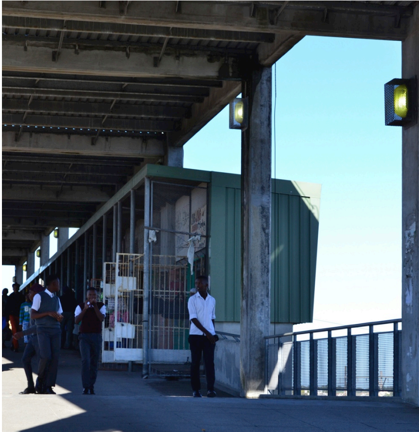
Figure 4.3 Philippi Station Pedestrian Bridge. The lightweight metal trading spaces contrast the robust concrete frame of the bridge. Photograph by author, 2012.
