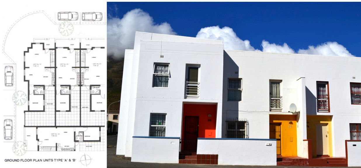
Figure 3.25 Pilot Project Corners. Corner units are set forward from the building line, as seen above in plan and photograph, in reference to the historic ‘elaboration of corners’ which was noted in the HIA. Left from Digest of South African Architecture 2004/2005. Right Photograph by author, 2012.
