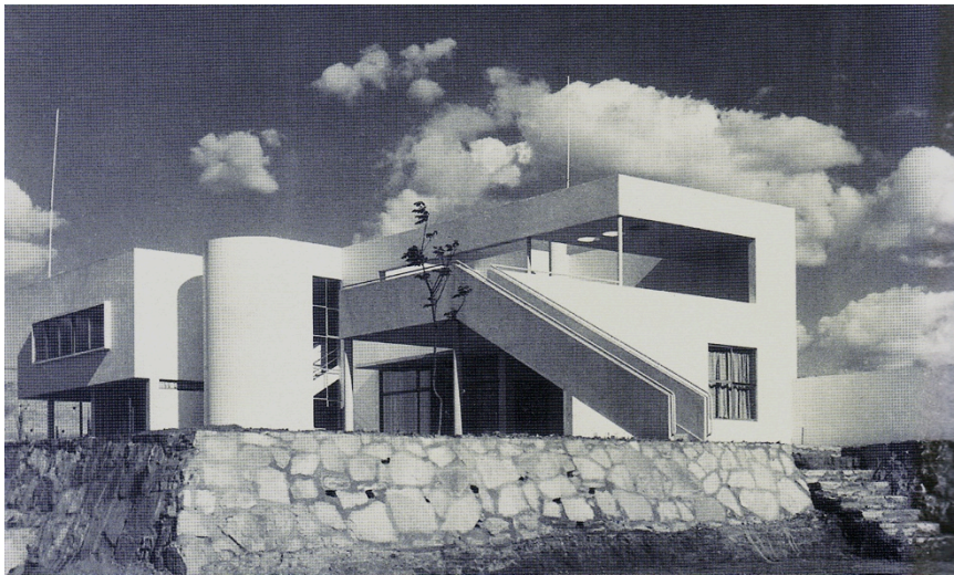
Figure 4.22 House Stern. The house illustrates the affinities with 'International Style' architecture, with its taught white skin, plastic forms, flat roof and horizontal windows and openings. From Herwitz 1998, 404.
