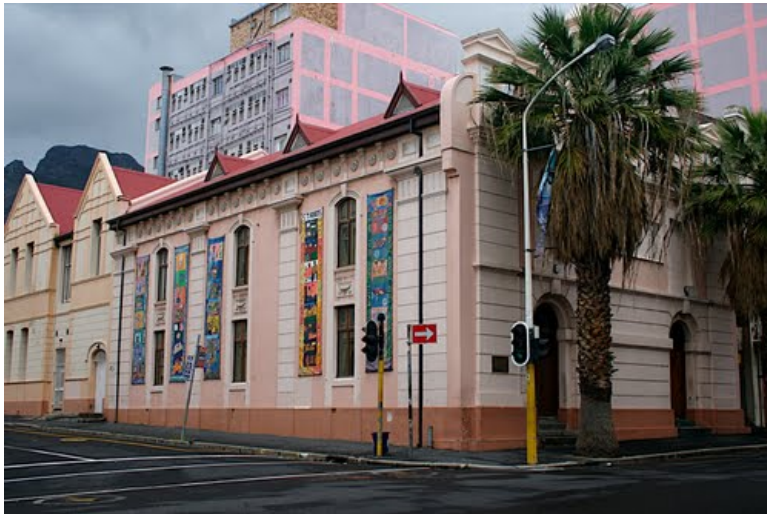
Figure 3.19 Methodist Church. The church, converted into the District Six Museum, is located on busy Buitenkant Street, just outside the former edges of District Six.
