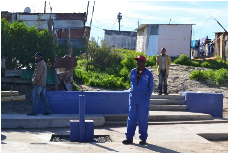
Figure 4.35 Khayelitsha Platform. Designed and constructed by University of Cape Town students, in 2012-2013, the platform uses a few features to accomplish a number of things: it negotiates a slope between rows of shacks where there is otherwise not a path, provides a water point, provides seating on the low walls, and clears out a space for gathering and activities. Photograph by author, 2013.
