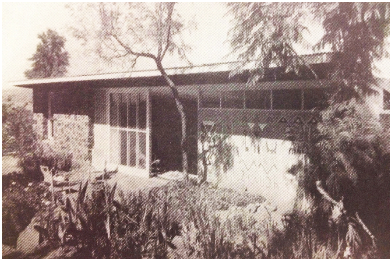
Figure 4.23 Farmhouse Stauch, by Hellmut Stauch, 1943. The ‘farmhouse’ reveals deep eaves and rustic stonework that visually and experientially tie the house to the locale. From Peters 1998.
