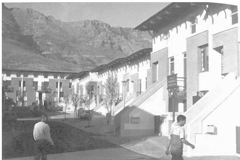
Figure 3.17 Springfield Terrace. The project by Headstart consisted of stacked flats organized around stoop-like front staircases, which met the ground at pedestrian-scaled courtyards that accommodated a small amount of parking. From Architecture SA Nov./Dec. 1993.
