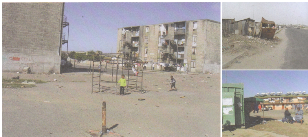
Figure 4.8. Images of neglect. Like Figure 4.6, these images were chosen by the leaders of the DPP to represent the types of spaces the program sought to intervene in. From Southworth 2010, 102.
