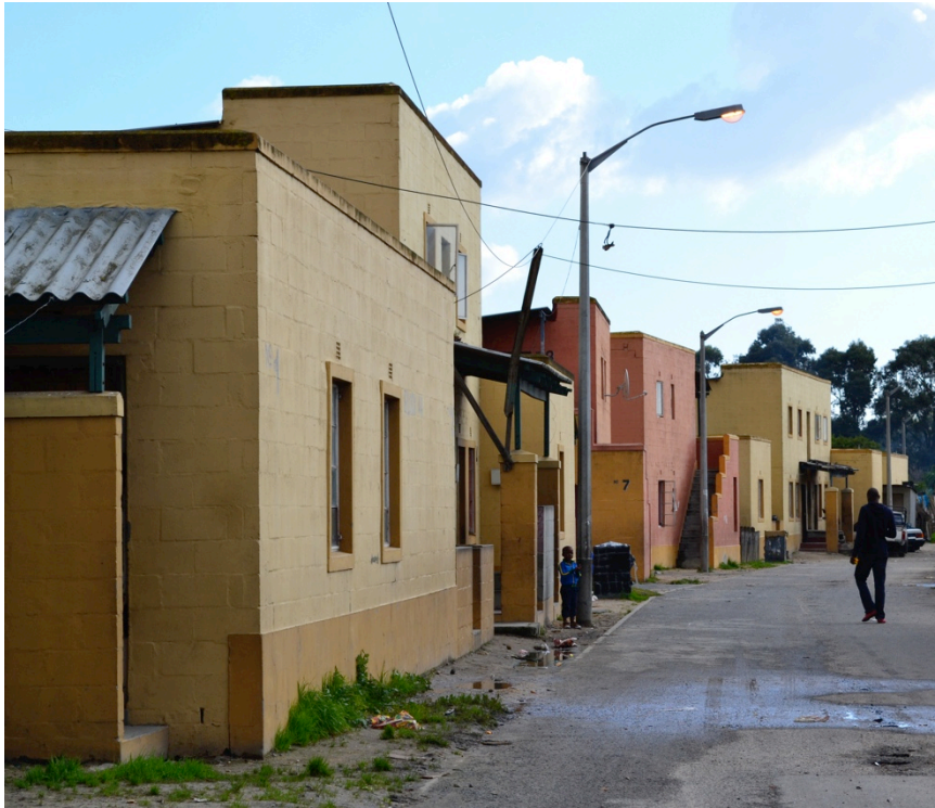
Figure 5.1 Nyanga Hostels Upgrades. The space immediately surrounding the upgraded hostels shows neglect, with dirt, weeds and trash where landscaping was intended. Photograph by author, 2012.
