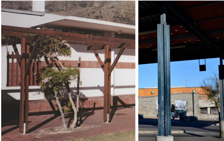
Figure 4.32 The ‘Cape Column’. Uytendogaardt’s trademark detail, in which two vertical members sandwich a horizontal or diagonal one, find echo in the columns of the PPTI taxi rank. Left Photo from Vio 2006; Right Photo by author, 2012.
