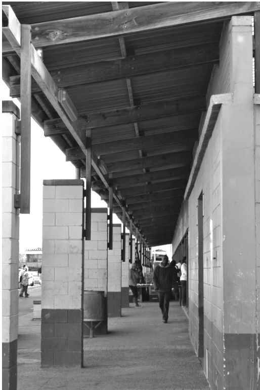
Figure 4.29 Trading Bay Building. Painted concrete block was the dominant material used at the level inhabited by the body. Photo by author, 2012.
