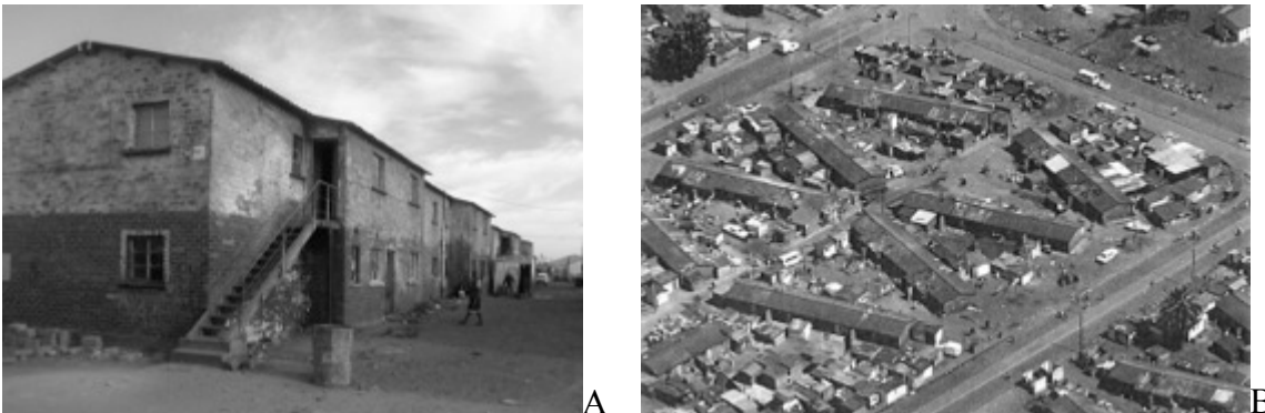
Figure 2.6 A row of hostels that had not yet been upgraded. The buildings were deteriorating but their appearance suggested that even when newly built, they would not have appeared much more hospitable, with uninsulated roofs and walls, and only minimal windows to allow in natural light. The space between the buildings was an undifferentiated expanse of dirt, that did not mark graduated degrees of public and private space, and did not offer support for daily activities such as washing or congregating. Photographs courtesy of Architects Associated.
