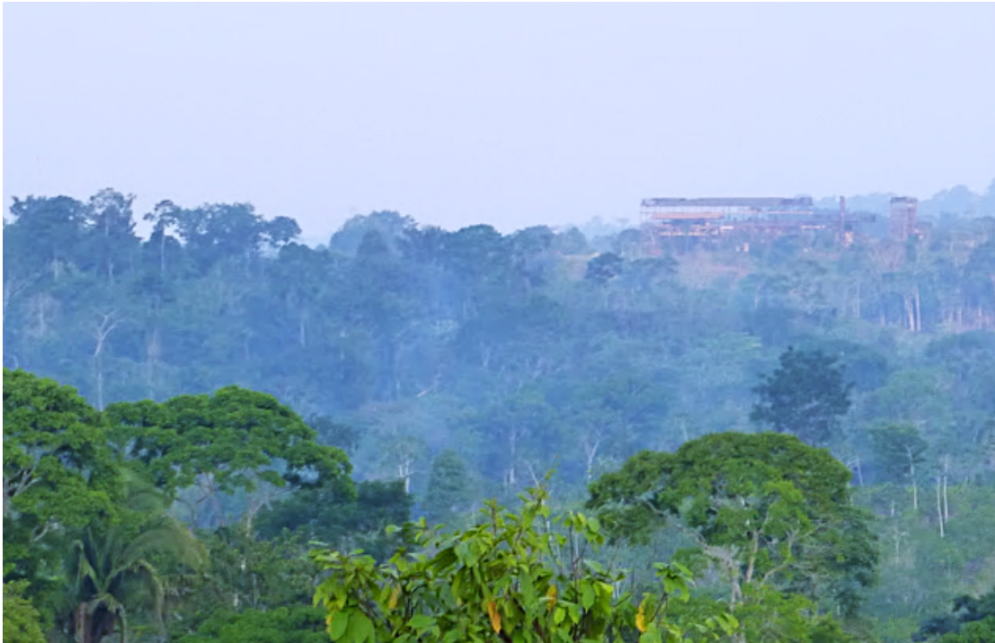
Figure 1.12 The ruined Abraham Lincoln Sugarcane Agroindustry Project (PACAL) mill-refinery, at distance of 3 kilometers from side road kilometer 95 south. Photograph by author.
