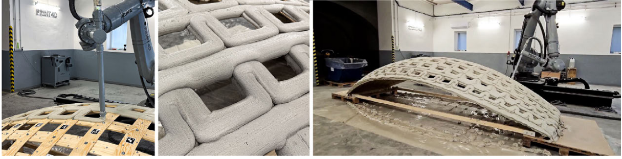
Figure 12: Conformal 3D printing process showing multi-axis platform maintaining perpendicular nozzle orientation for uniform concrete distribution, creating hybrid gridshell structure for wide-span construction.
