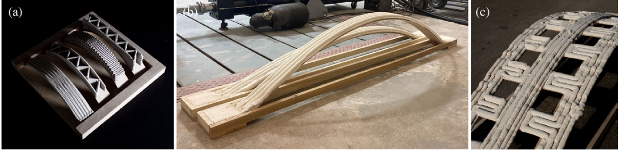
Figure 6: Small-scale conformal 3D printing experiments on bending-active formwork: (a) toolpath patterns on single strip, (b) concrete printing on single strips with varying curvature, and (c) multi-strip gridshell configuration.
