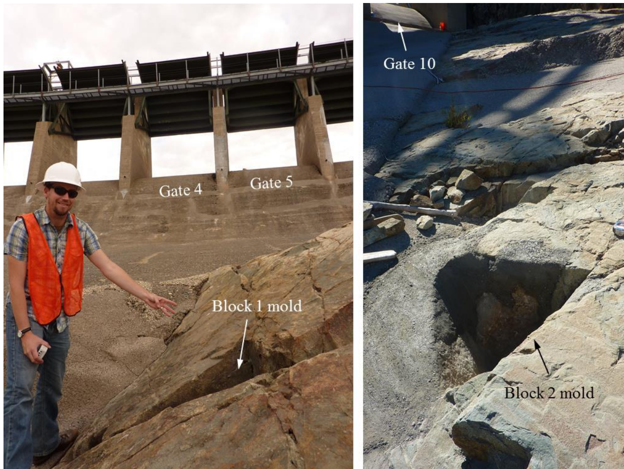
Figure 3-11. Tetrahedral molds for artificial rock blocks at Spaulding Dam No. 2. Note concrete added to Block 2 mold to provide continuity of the free face when the block is installed.
