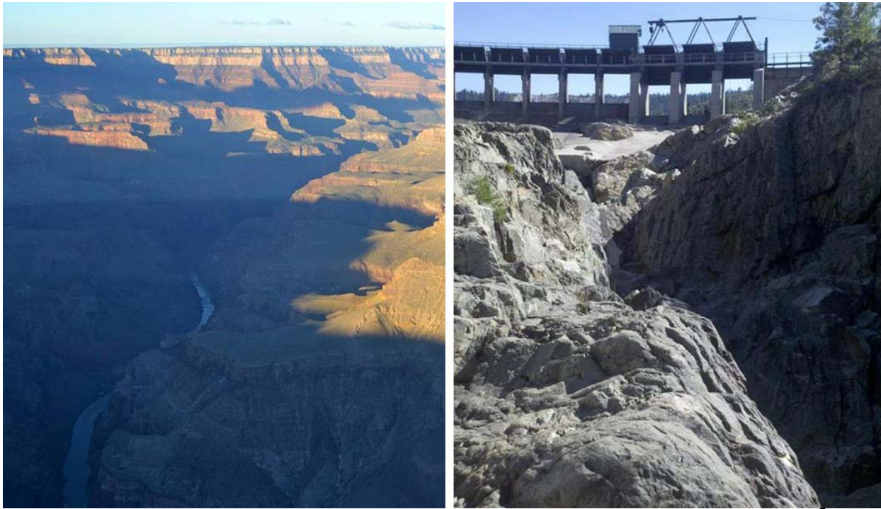
Figure 1-1. Erosion of Grand Canyon (left) by Colorado River over geologic time – O(10^7) years) (National Park Service 2015) and slot canyon (right) at Spaulding Dam in Northern California by reservoir spills over human time – O(10^1-10^2) years).
