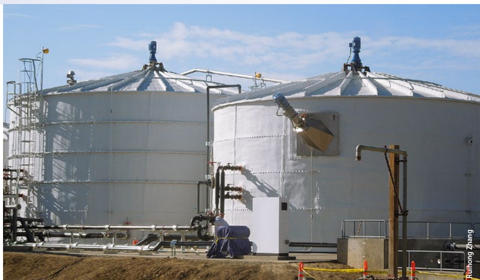
On the UC Davis campus, anaerobic digesters break down food waste and manure and generate biogas.
