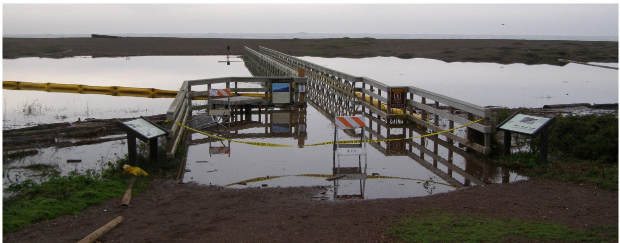
Fig. 4-5. Rodeo Lagoon was deeper than usual in this picture taken 09 January 2008, flooding the pedestrian bridge to Rodeo Beach. The yellow booms are a response to the Cosco Busan oil spill of 07 November 2007, which reached Rodeo Beach.
