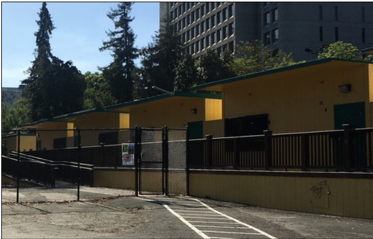
Figure 4: The New Temporary Mosswood Recreation Center.
