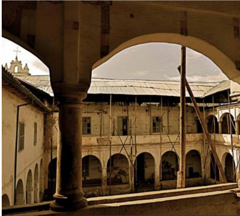
Figure 1.9. Former quarters of Convent Santa Clara la Real -under repair. Photograph of the Escuela Taller of Boyacá. 2013. Tunja, Casa Taller Boyacá.
