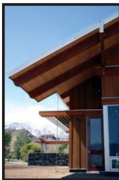
Figure 1. The design team included light-shelves and sun shades, highly reflective roofing, and fenestration that minimizes heat gain and loss and maximizes views of Mt. Whitney. (Photo: Bill Hustace)
