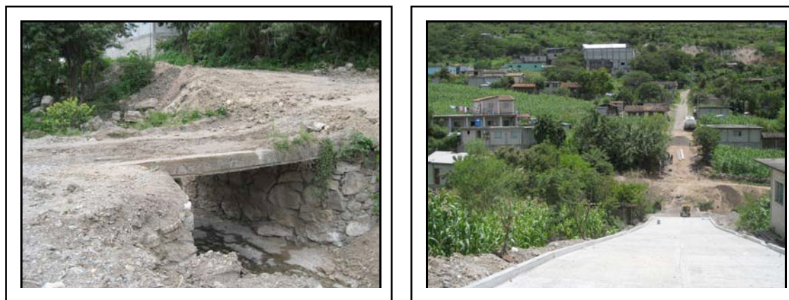
Image 3.1: Bridge in San Miguel Tlacotepec
